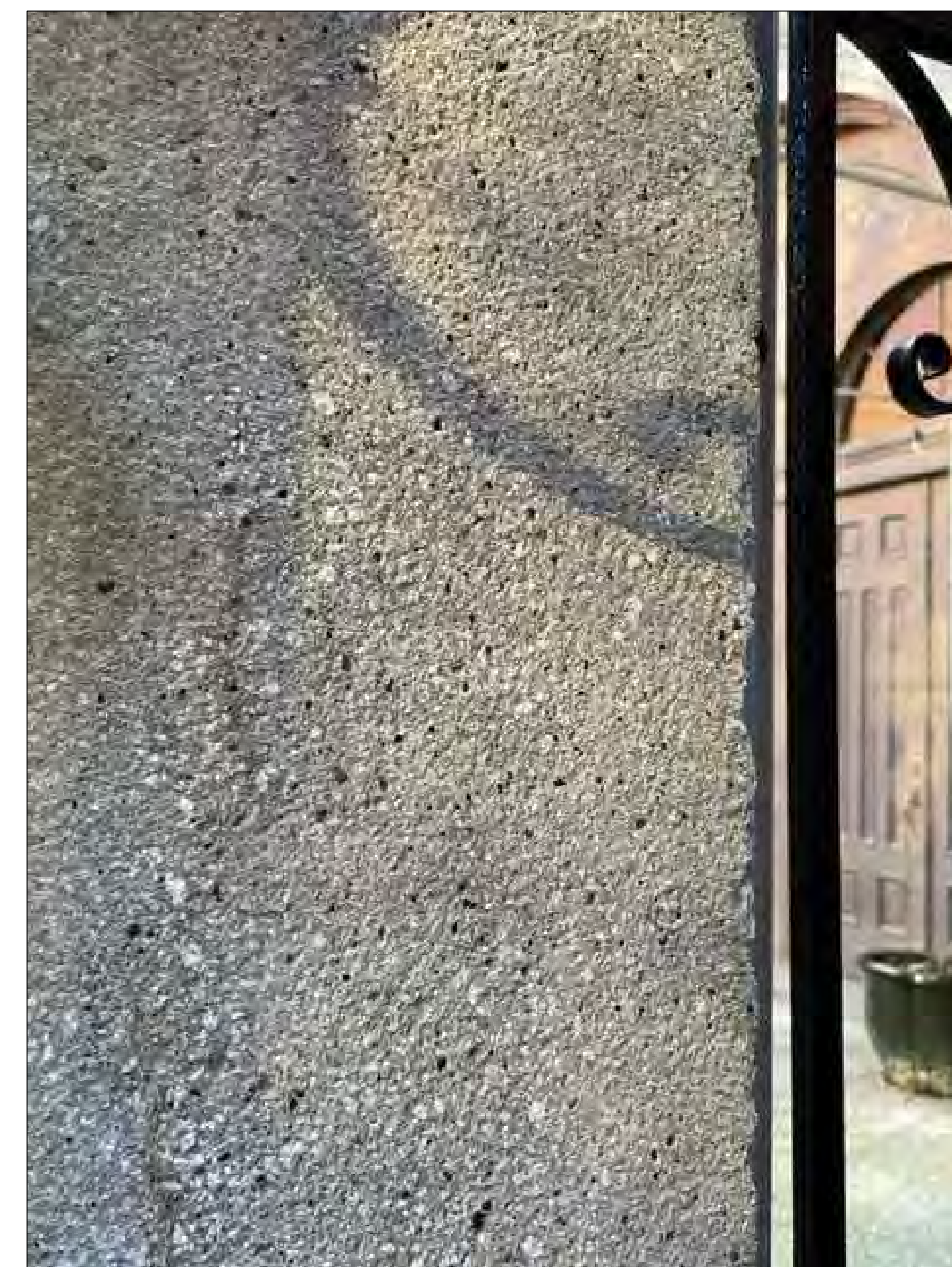
3 BUSH-HAMMERED WEST SURFACE OF PIER 'E'
