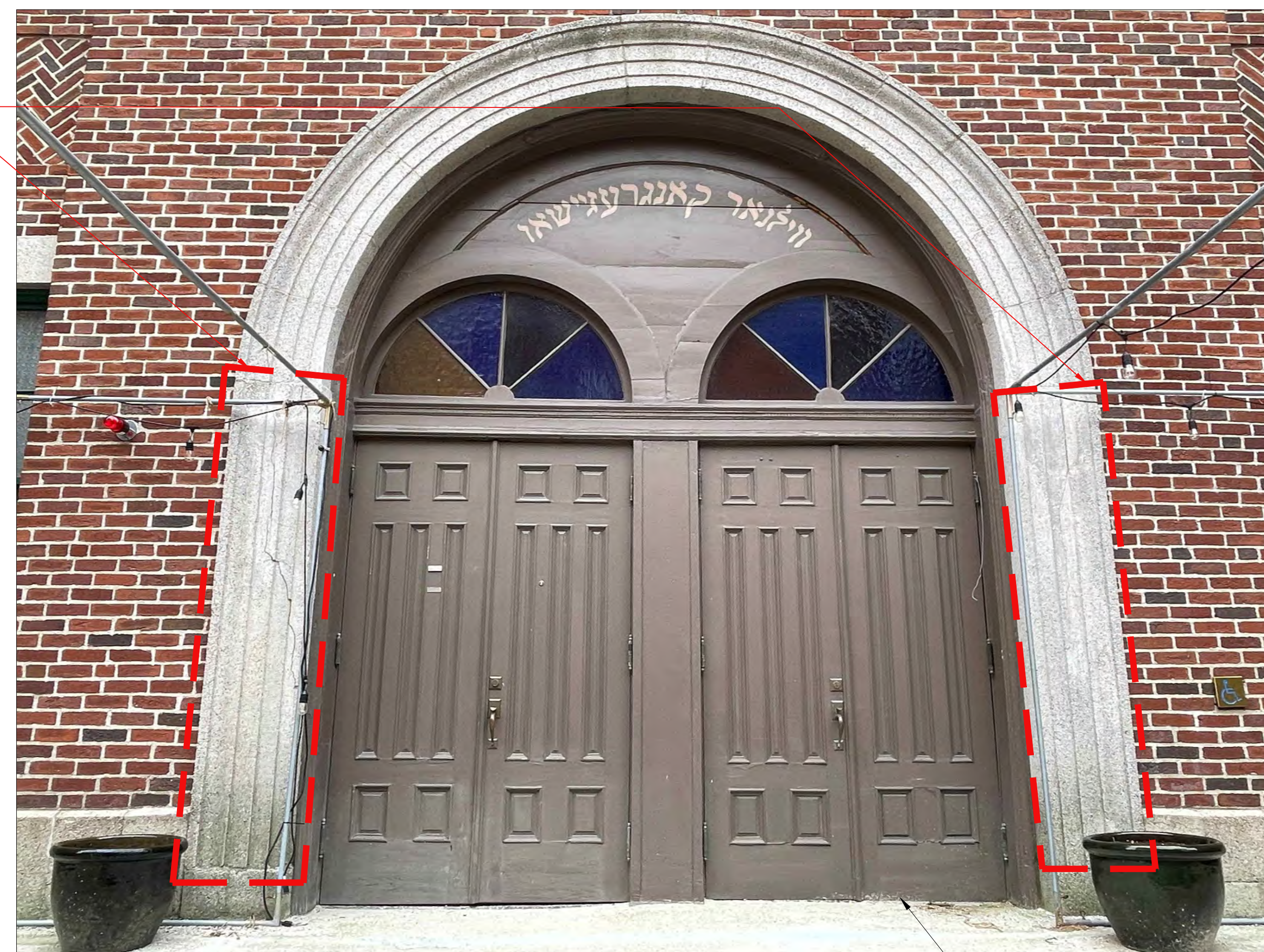
5 EXISTING ENTRY DOORS
