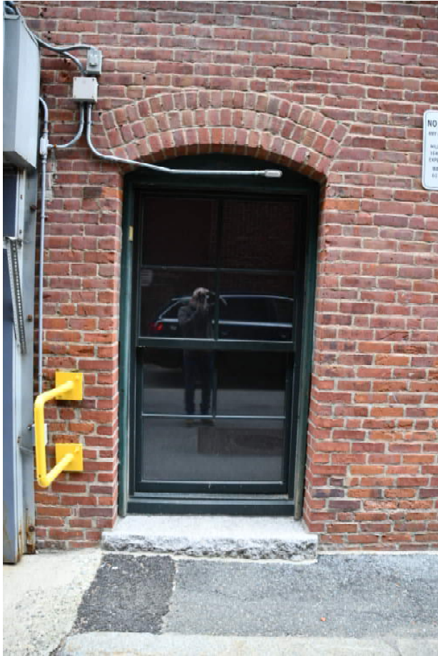
Existing wood trim surrounding the aluminum window systems.
