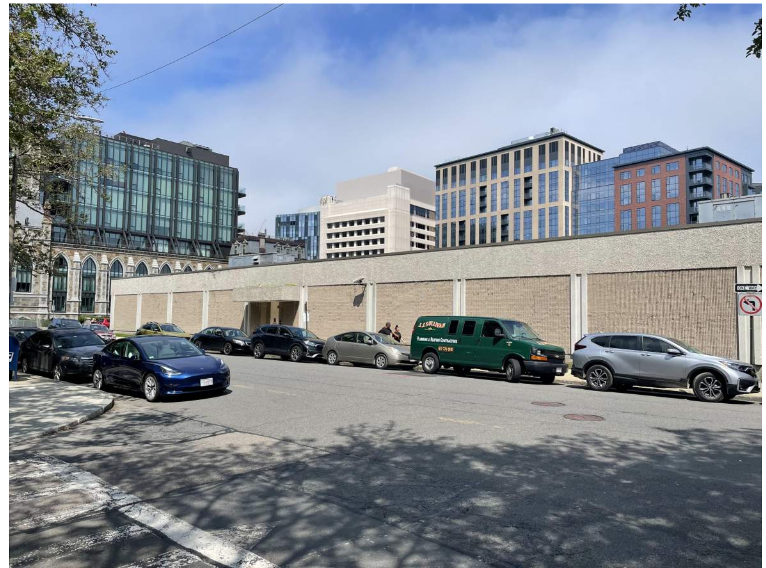
Proposed View within the Protection Area on Shawmut Ave (5).
