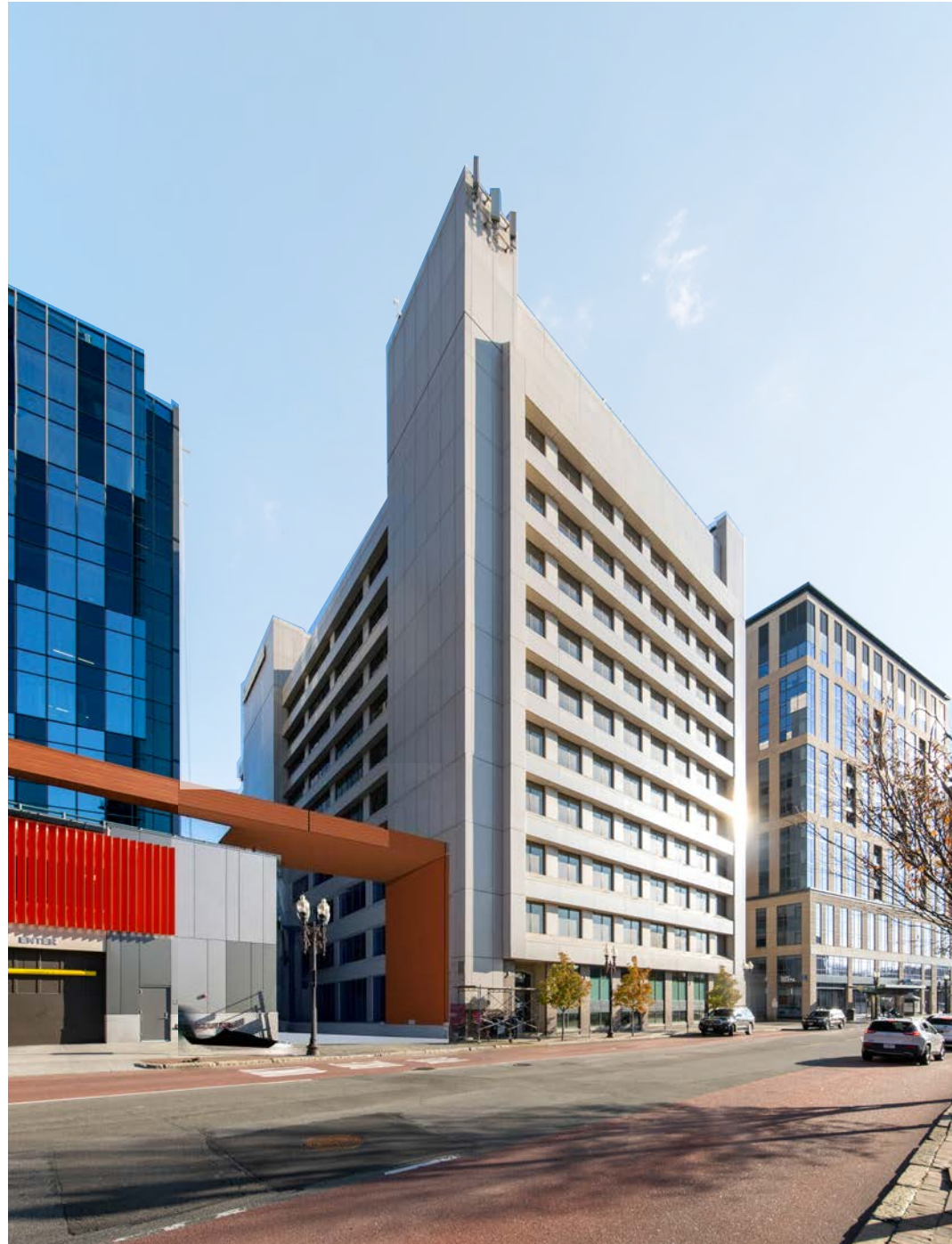
Existing Street Level View from the North West on Washington Street
