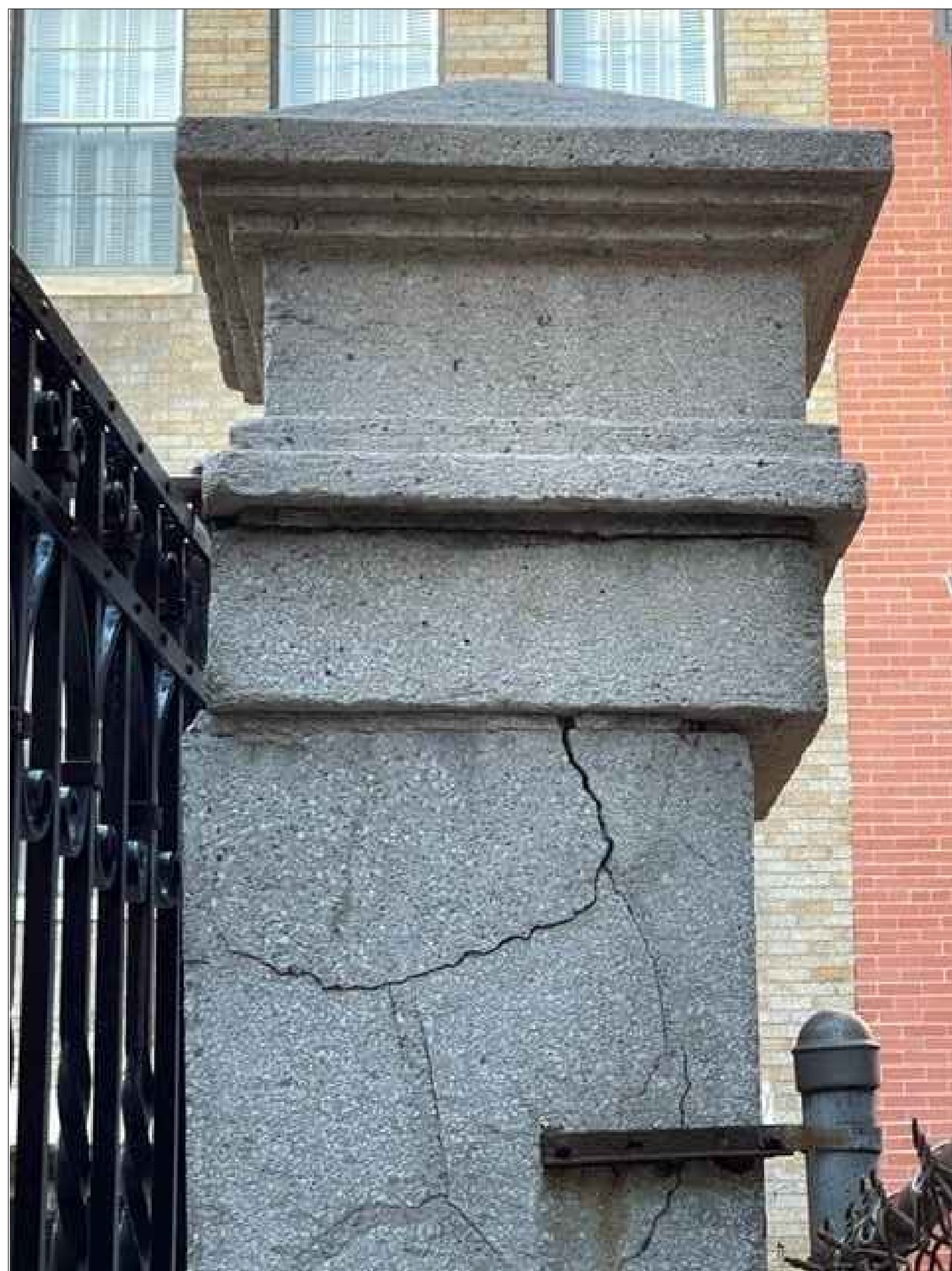
1 CLOSE-UP OF UPPER SOUTH SIDE OF PIER 'A' THIS IS WHERE SAMPLES WERE TAKEN; SEE SHEET A-10.
