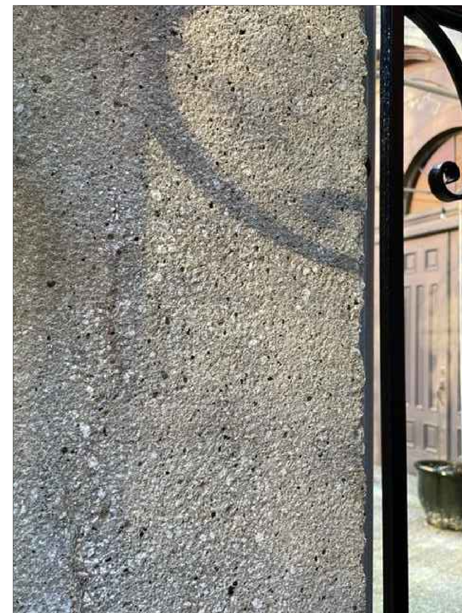
3 BUSH-HAMMERED WEST SURFACE OF PIER 'E'
