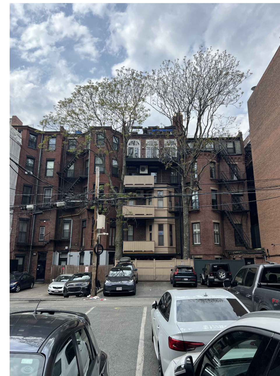
④ PHOTO VIA PUBLIC ALLEY 432
