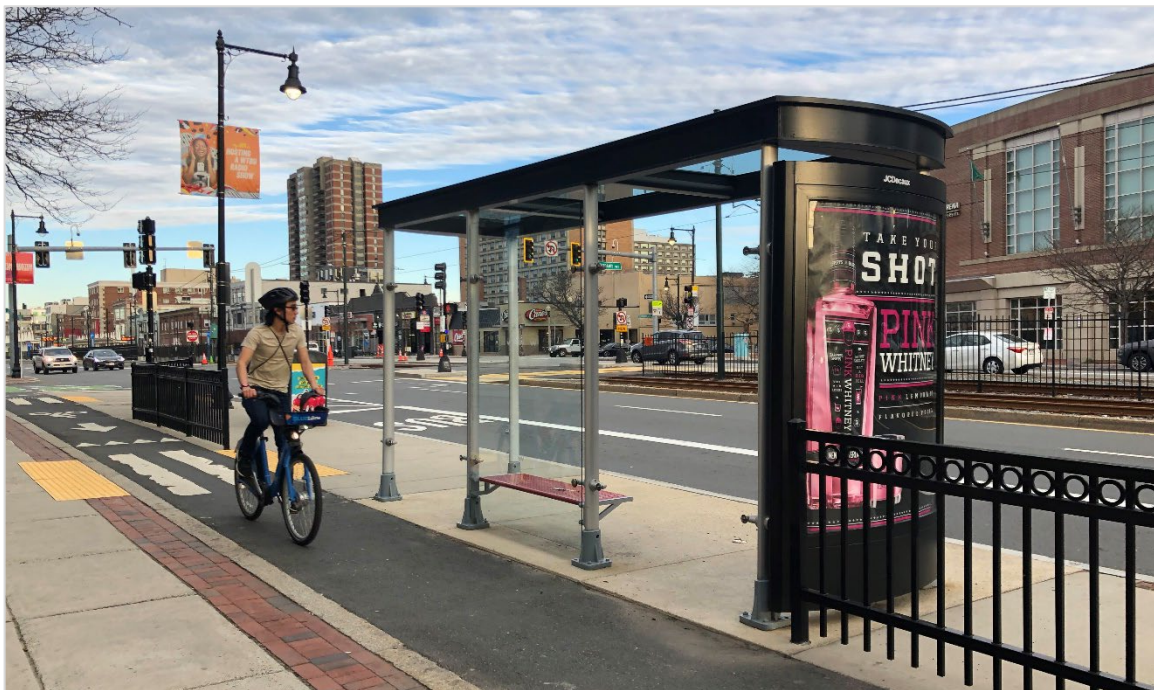
A person biking in a protected bicycle lane next to a floating bus stop on Commonwealth Avenue eastbound. Image source: Nelson\Nygaard.
