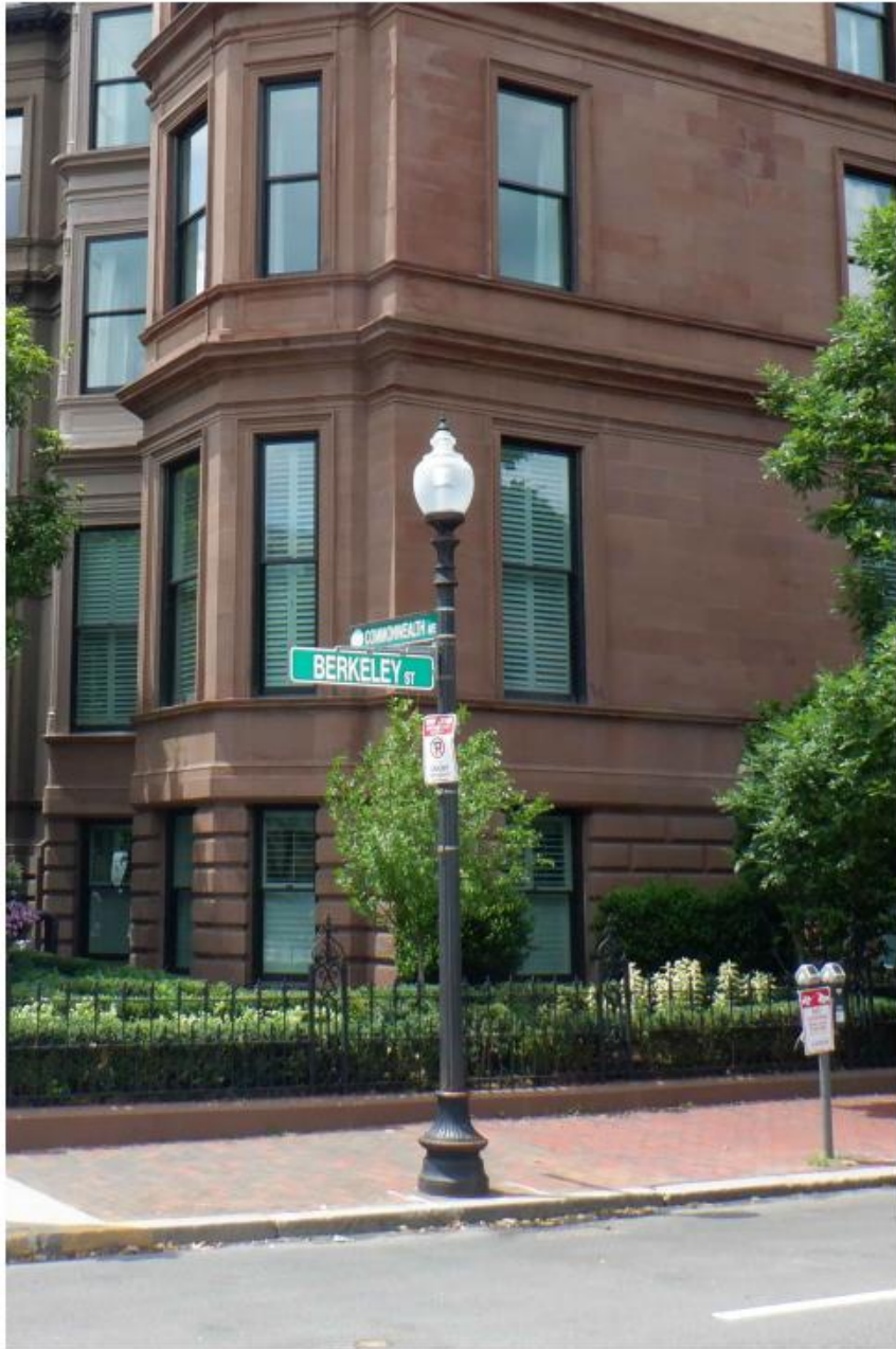
EXISTING PHOTOGRAPHIC VIEW
