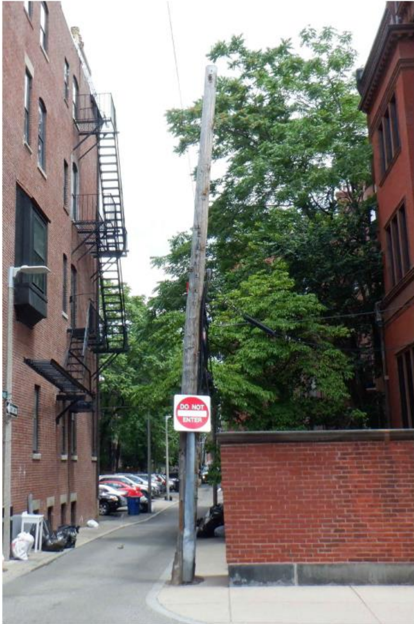
EXISTING PHOTOGRAPHIC VIEW
