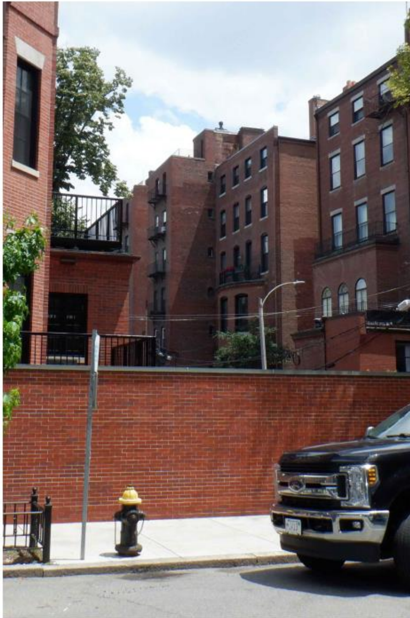
EXISTING PHOTOGRAPHIC VIEW
