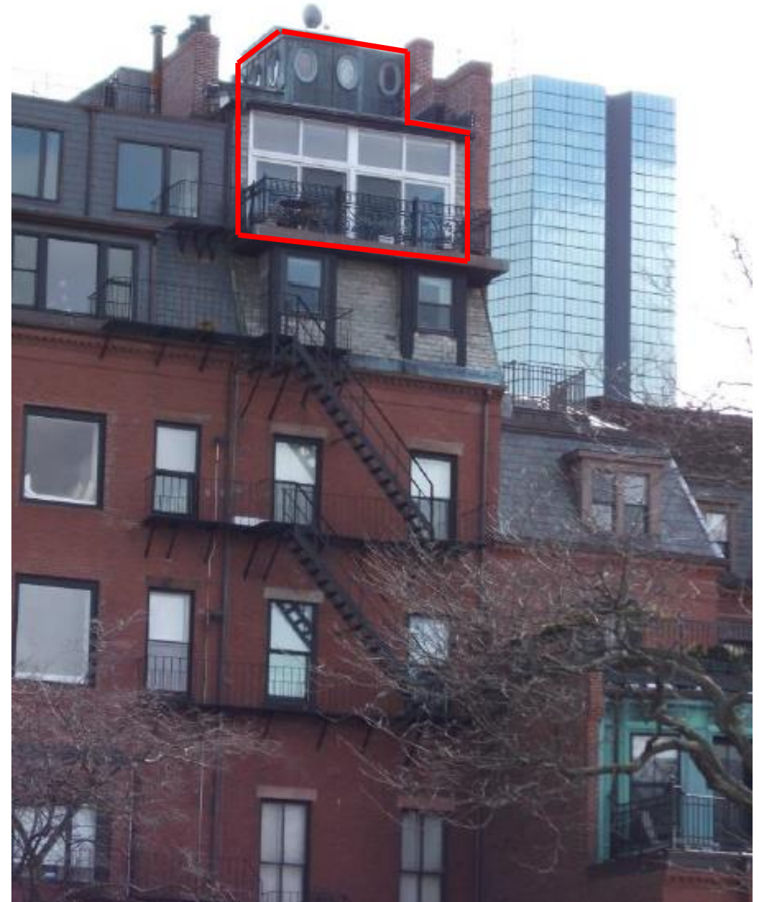
Red outline demarcates posterior sliding doors of PH R to be replaced. This is a head-on view.
