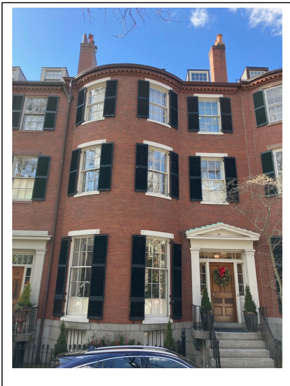
Front view of 14 Louisburg Square
