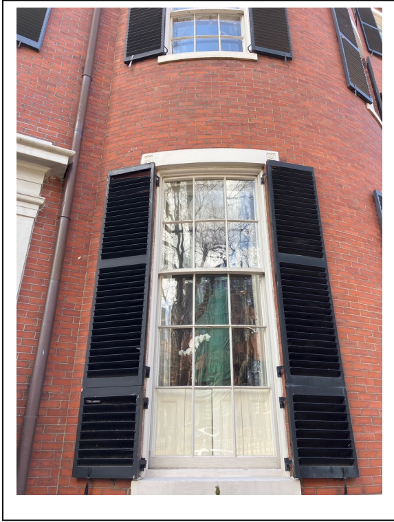
Close up of window shutters to be replaced
