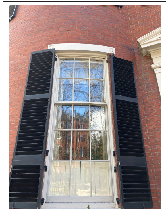
Close up of window shutters to be replaced
