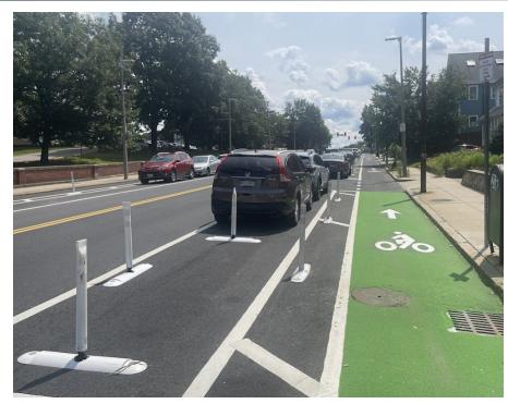
Above: example of a street design project using quick build materials. The photo shows flexible plastic bollards and striping. Location: South Huntington Ave, Jamaica Plain
