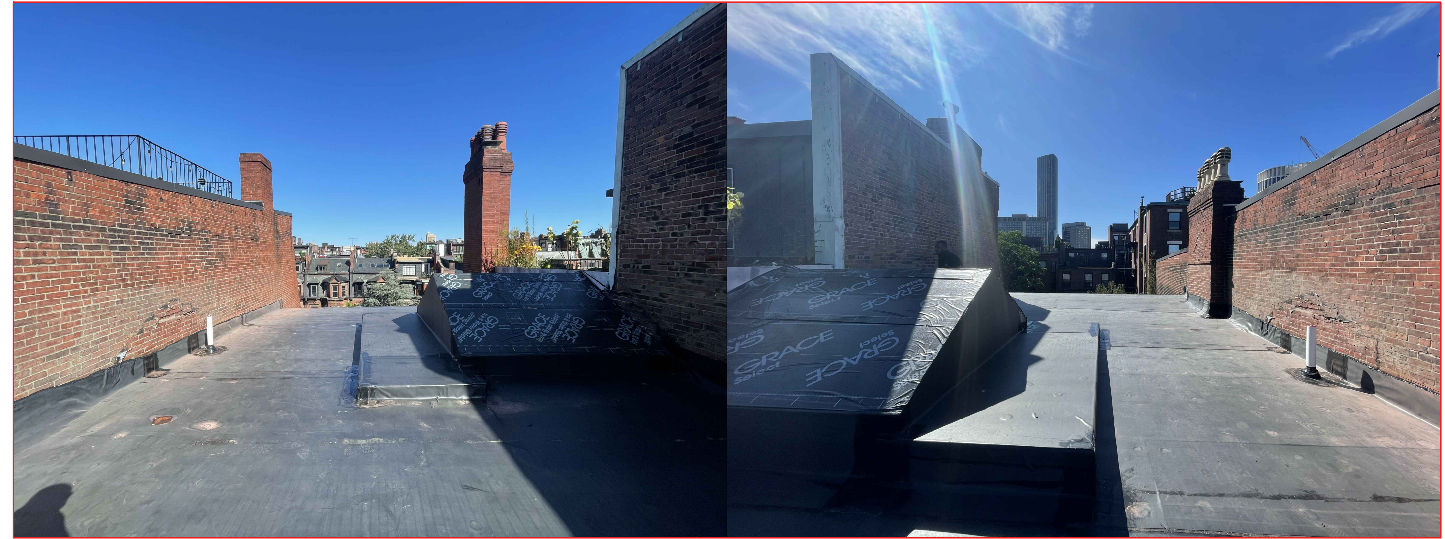
EXISTING CONDITION SKYLIGHT / ROOF HATCH
