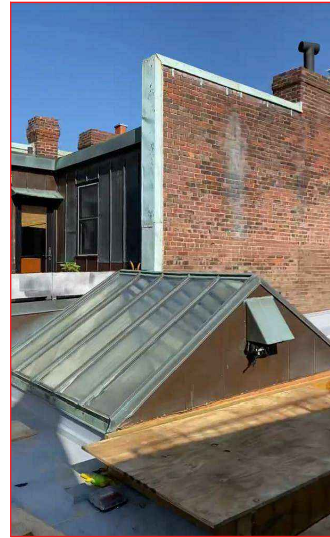
PREVIOUS CONDITION SKYLIGHT / ROOF HATCH
