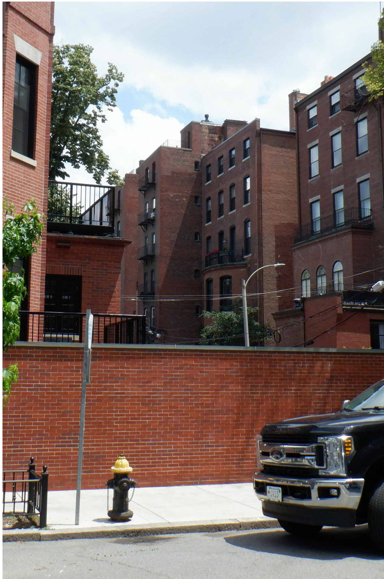
EXISTING PHOTOGRAPHIC VIEW
