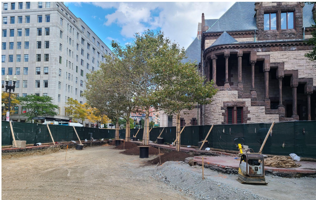
4 mature London Plane trees by Trinity Church were discovered to have too many large roots to install the pavement and tree grates around them. So they will breathe easier with a planter!
