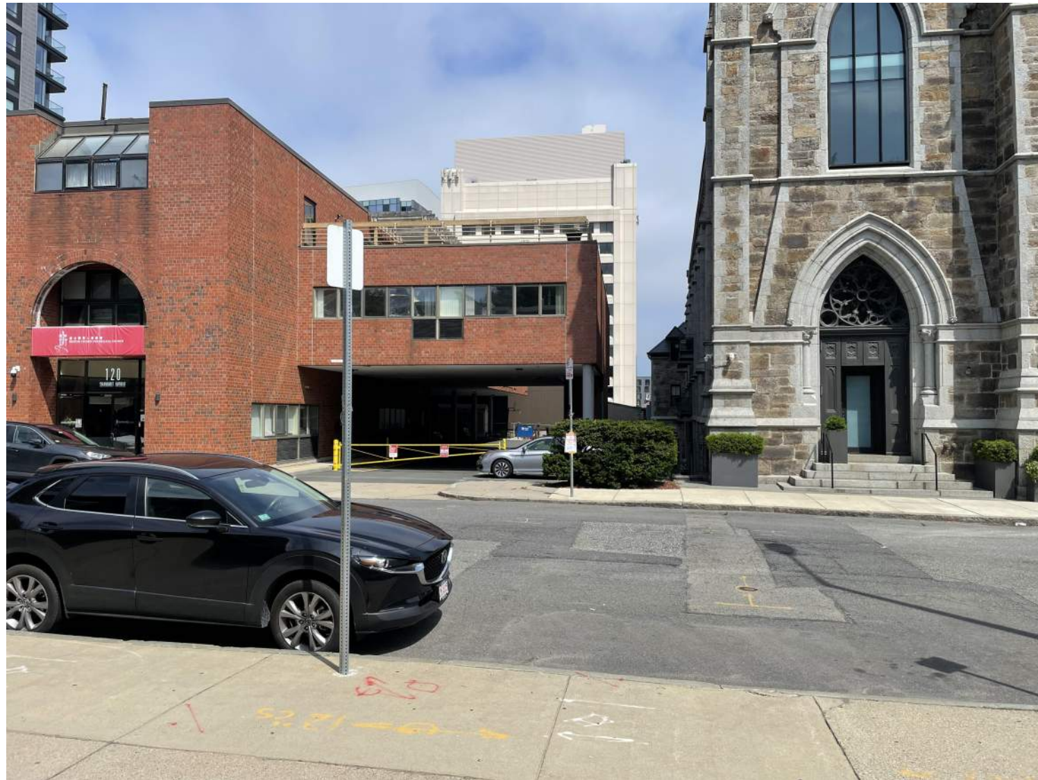
Proposed View within the Protection Area on Shawmut Ave (6).
