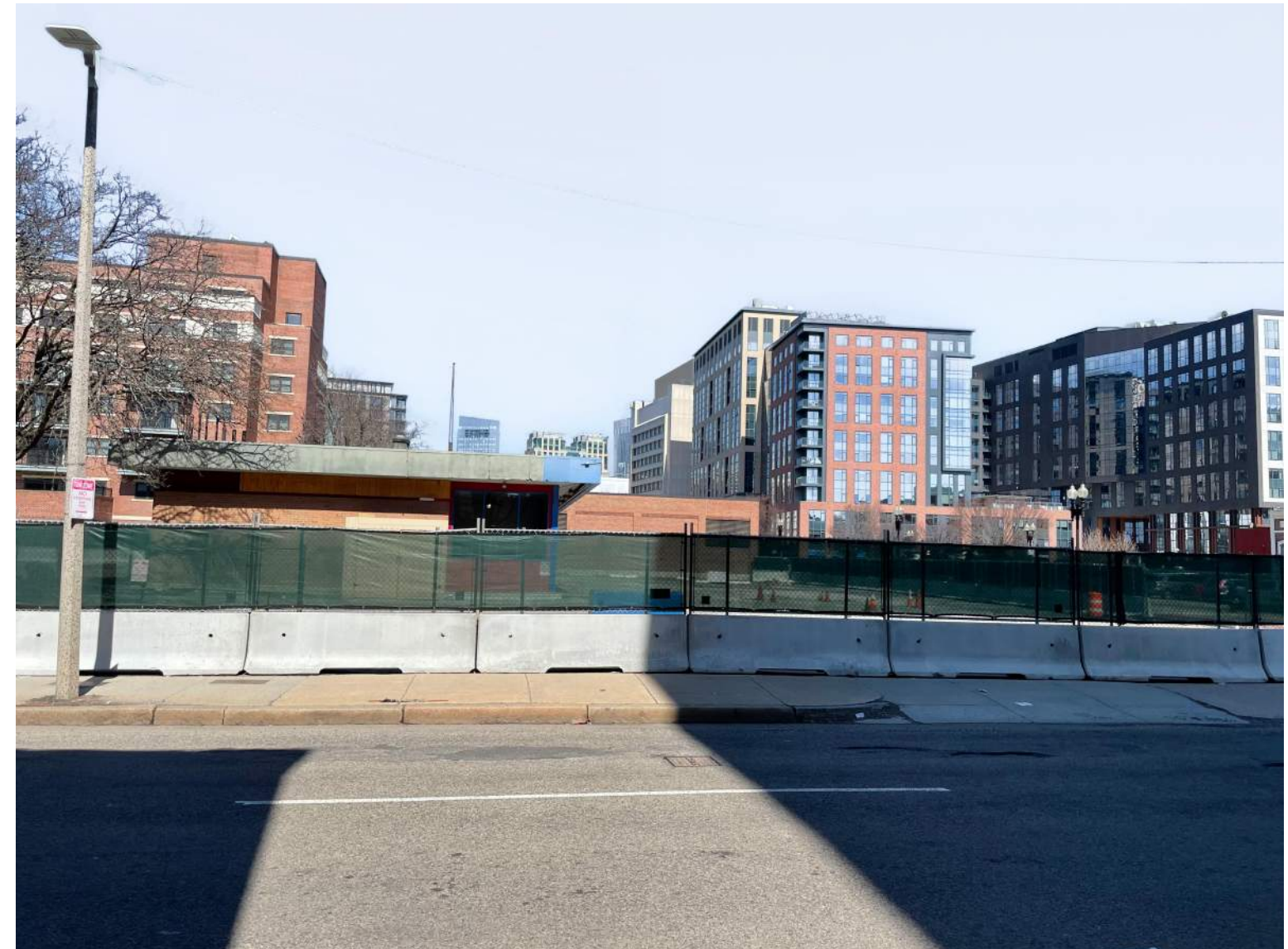
Proposed View at Landmark District Boundary on East Berkeley Street (3)
