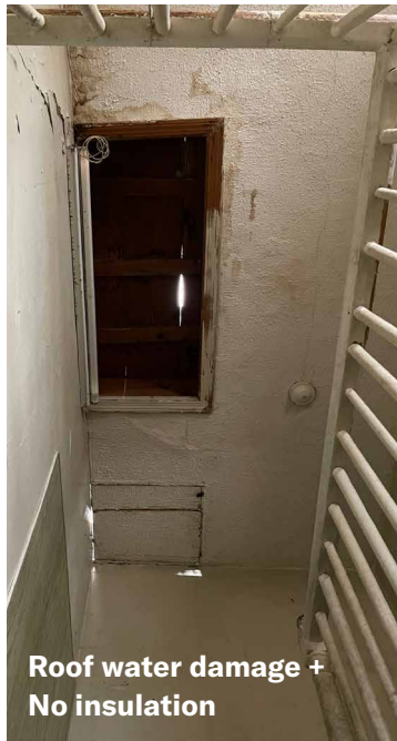
1st floor: damaged ceiling, water leakage
