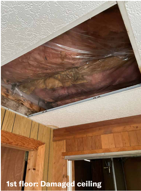
1st floor: damaged ceiling, water leakage
