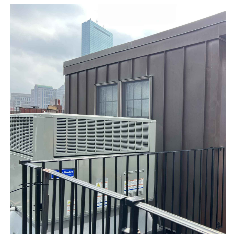
4 PHOTO VIA ROOF
