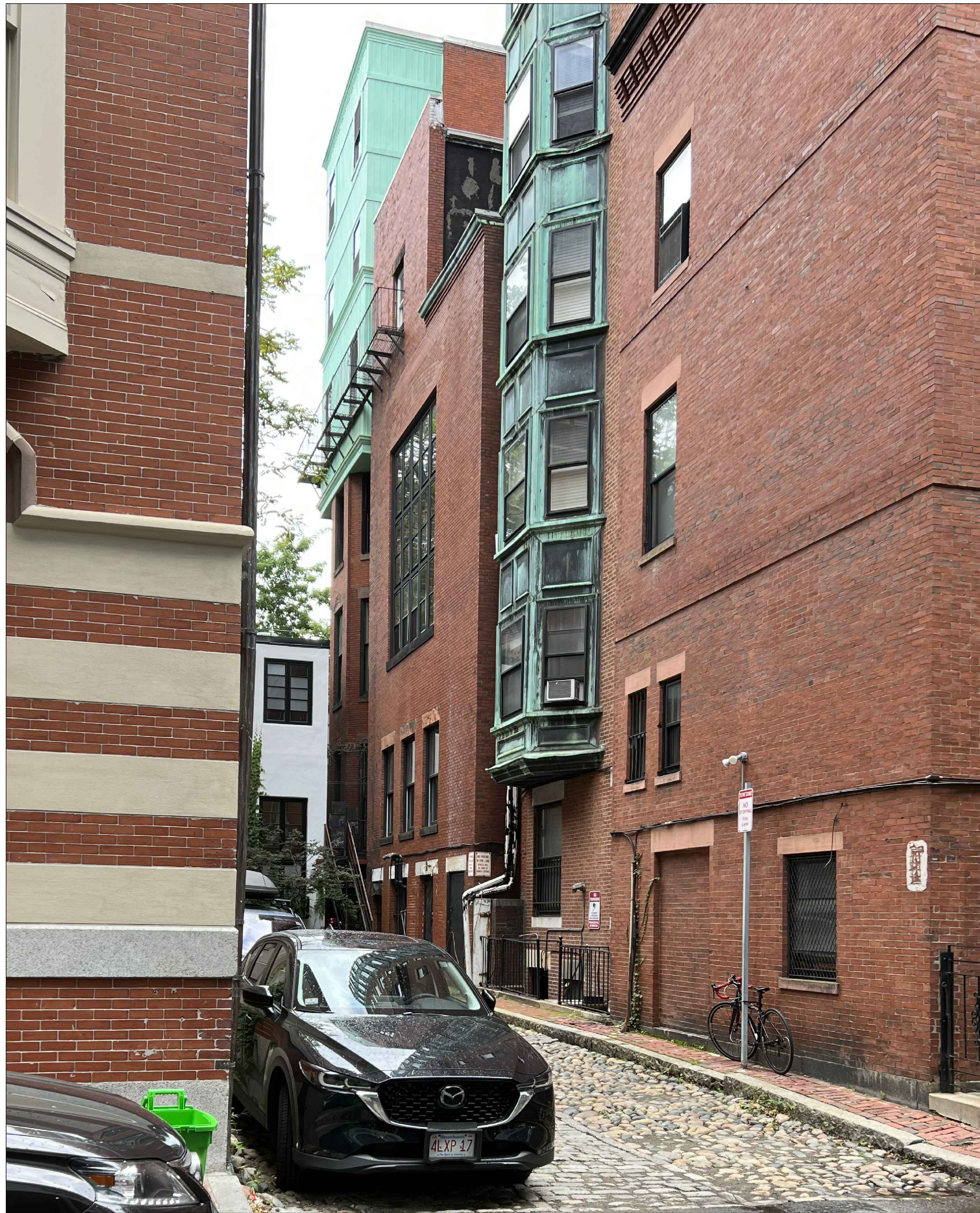
EXISTING VIEW FROM SPRUCE STREET
