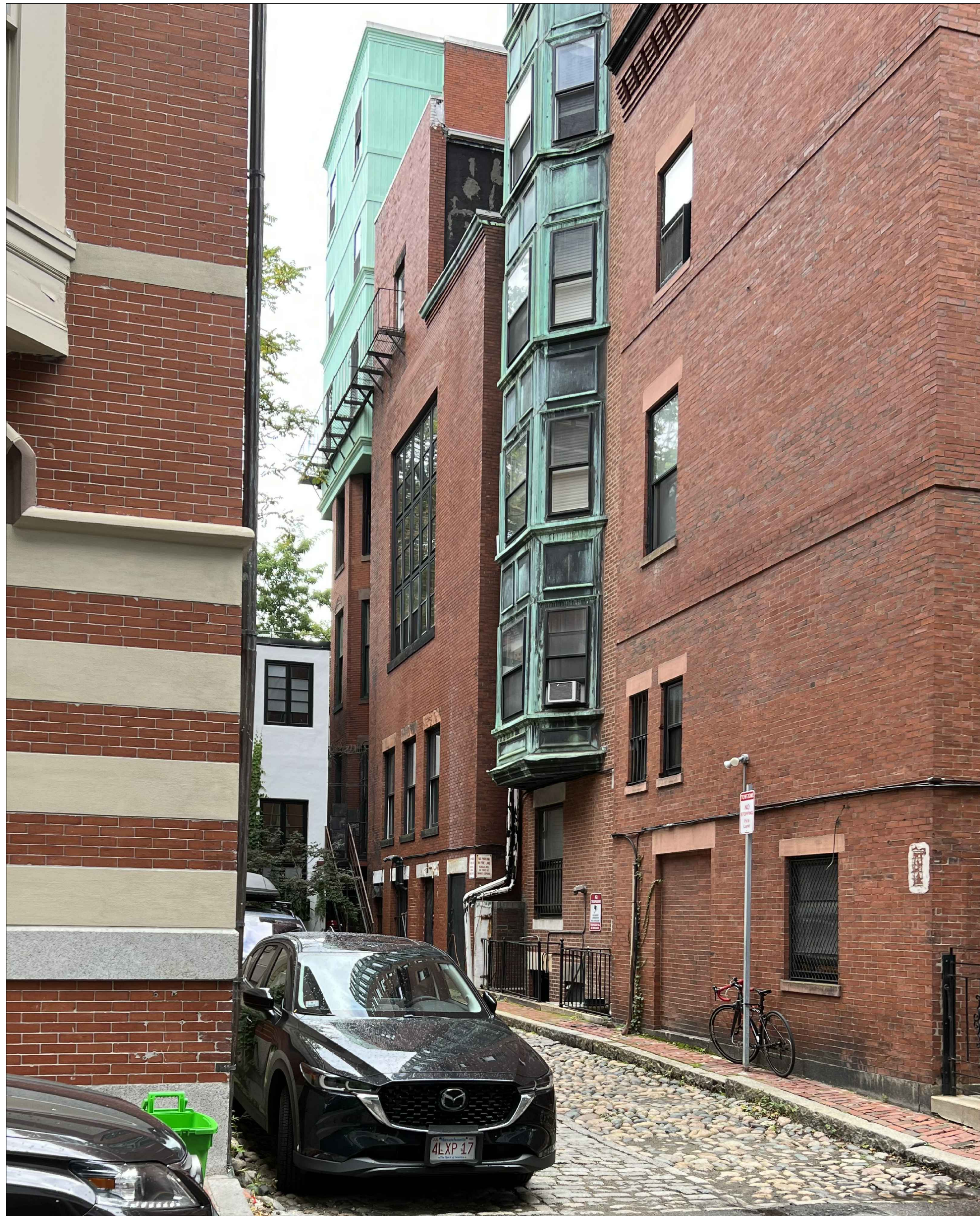
EXISTING VIEW FROM SPRUCE STREET
