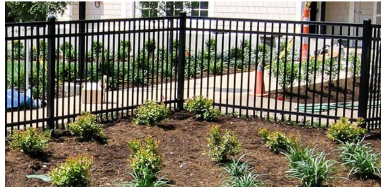
36" Ornamental Fence – to be mesh screen as shown on the left, OR simple aluminum fence as above, depending on budget
