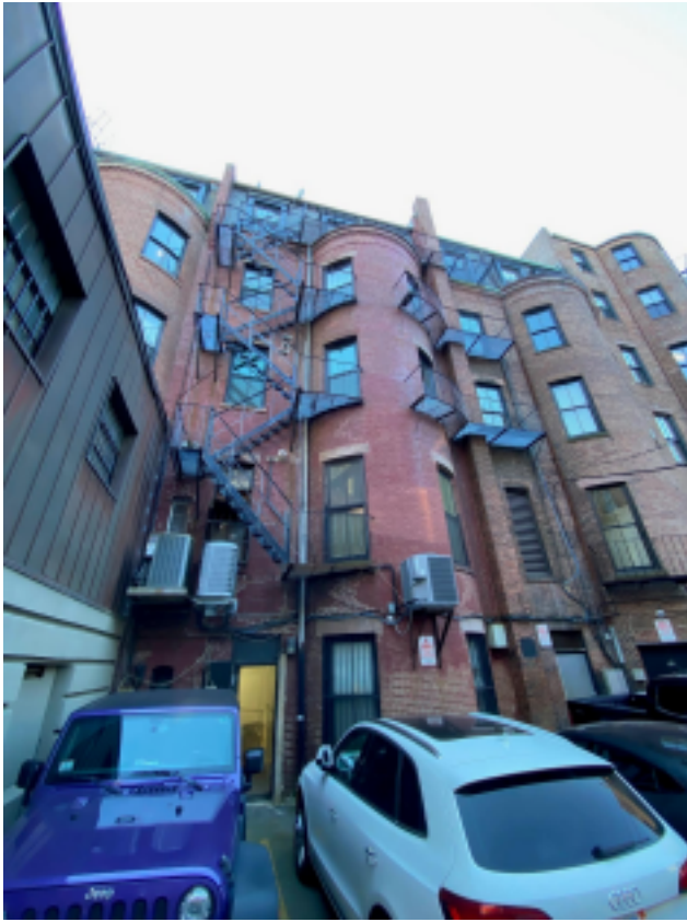
121 Newbury Street: Back Bay Review Alterations to Rear Elevation Existing Condition Photographs - Rear Alley
