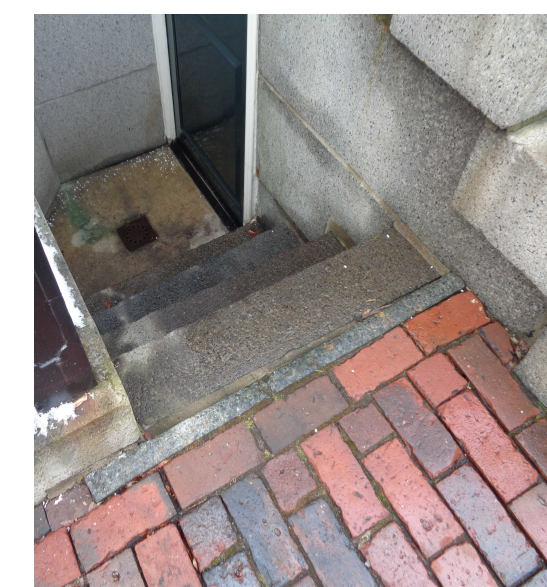
IMAGE OF EXISTING LOWER ENTRY STAIRS AT 10 LOUISBURG SQUARE TAKEN ON 1/19/24
