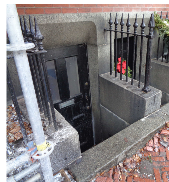
IMAGE OF EXISTING LOWER ENTRY STAIRS AT 4 LOUISBURG SQUARE TAKEN ON 1/19/24
