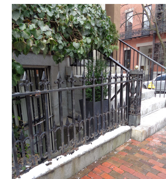
IMAGE OF EXISTING LOWER ENTRY STAIRS AT 22 LOUISBURG SQUARE TAKEN ON 1/19/24
