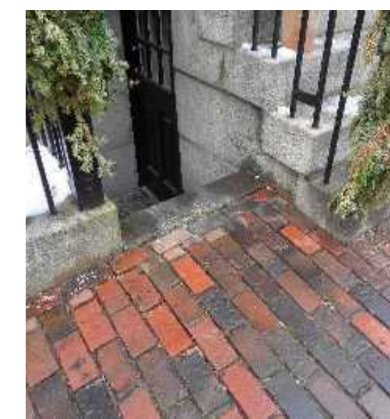
IMAGE OF EXISTING LOWER ENTRY STAIRS AT 12 LOUISBURG SQUARE TAKEN ON 1/19/24
