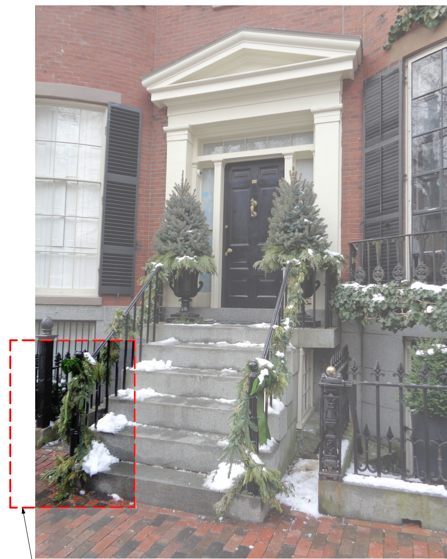
DASHED LINE DENOTES LIMIT OF PROPOSED WORK VIEW OF 20 LOUISBURG SQUARE ENTRY FROM PINCKNEY STREET
