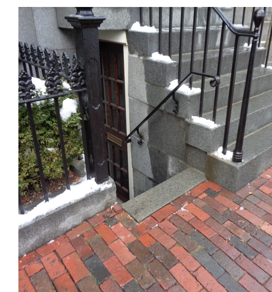
IMAGE OF EXISTING LOWER ENTRY STAIRS AT 16 LOUISBURG SQUARE TAKEN ON 1/19/24
