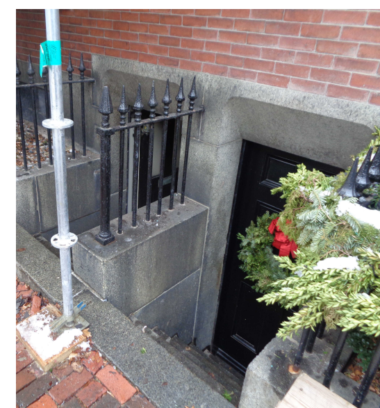
IMAGE OF EXISTING LOWER ENTRY STAIRS AT 6 LOUISBURG SQUARE TAKEN ON 1/19/24
