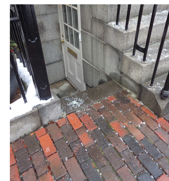
IMAGE OF EXISTING LOWER ENTRY STAIRS AT 14 LOUISBURG SQUARE TAKEN ON 1/19/24
