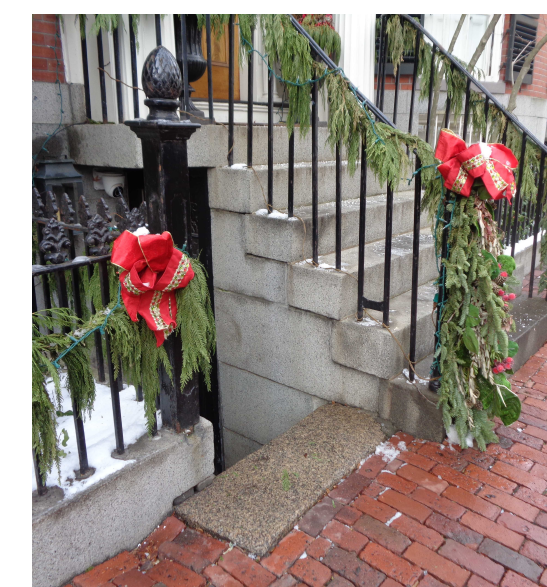
IMAGE OF EXISTING LOWER ENTRY STAIRS AT 8 LOUISBURG SQUARE TAKEN ON 1/19/24
