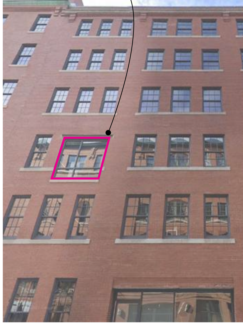
20 Channel Center - Channel Center Facade
