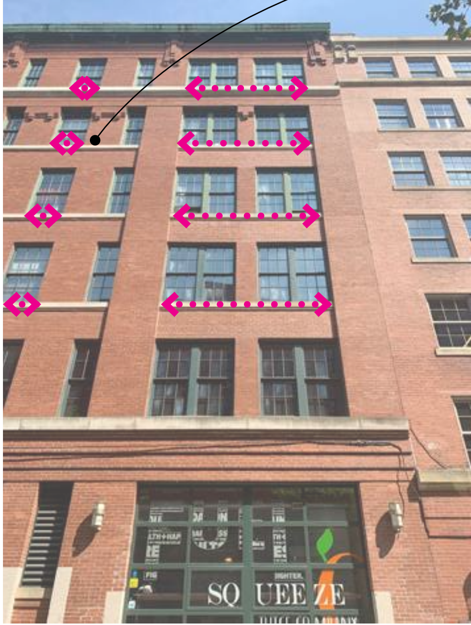
15 Channel Center - Channel Center Facade
