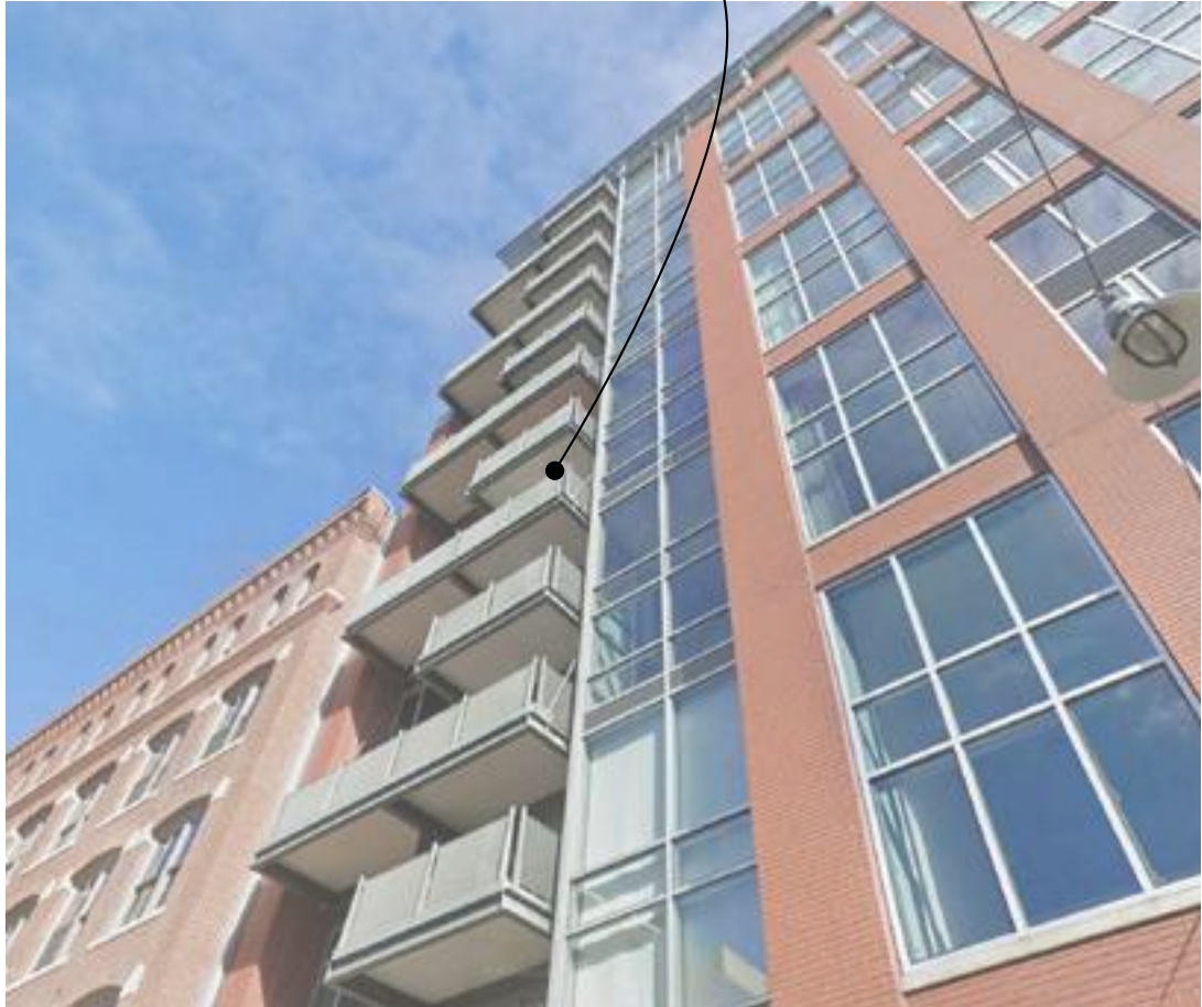
25 Channel Center - Channel Center Facade
