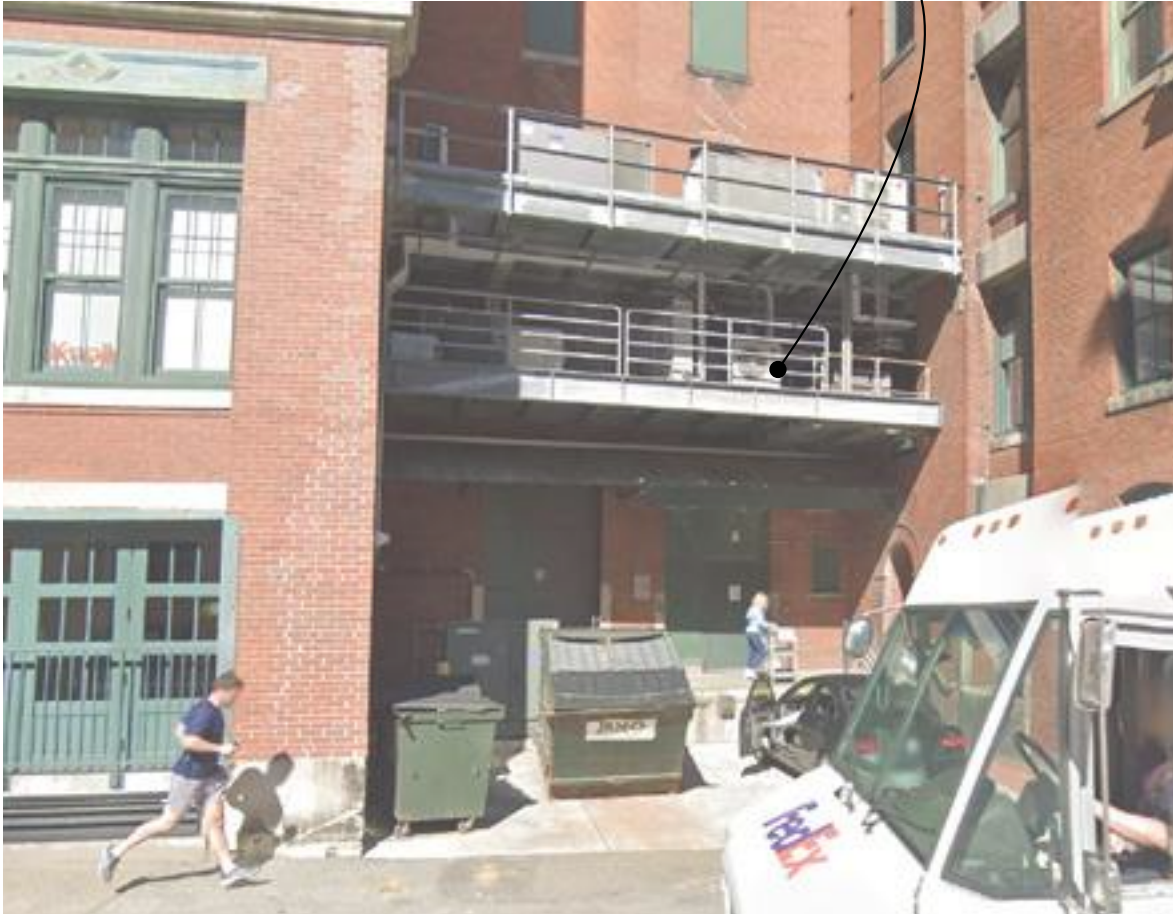
273 + 281 Summer Street - Melcher Street Facade
