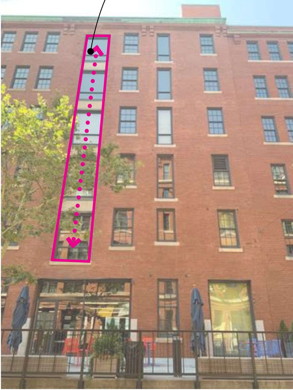
20 Channel Center - Channel Center Facade
