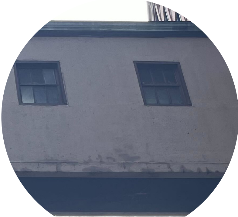
STUCCO REPAIR & REPAINTING
