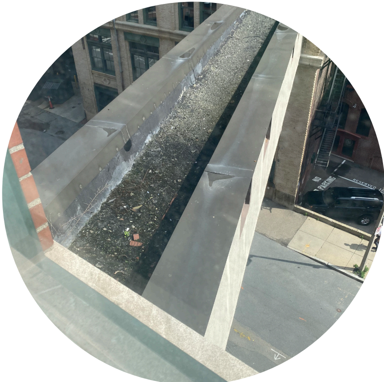
ROOF REPAIR & REPLACEMENT
