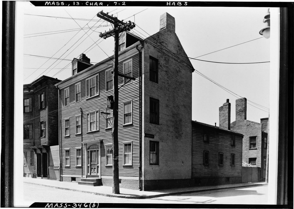
Figure 28. A 1933 photograph of the Apollos Field House, looking northwest.
