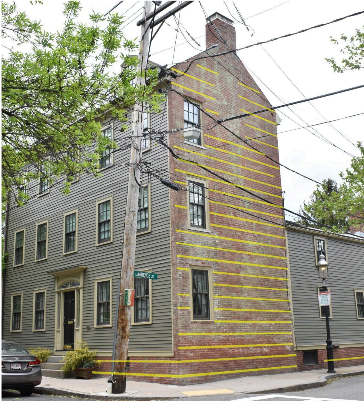
Figure 21. 30 Union St.'s east-facing brick end wall with header rows highlighted to illustrate inconsistencies in construction. Deviating header intervals and omission at the chimney stack suggest that the house was originally two or two-and-one-half stories in height.
