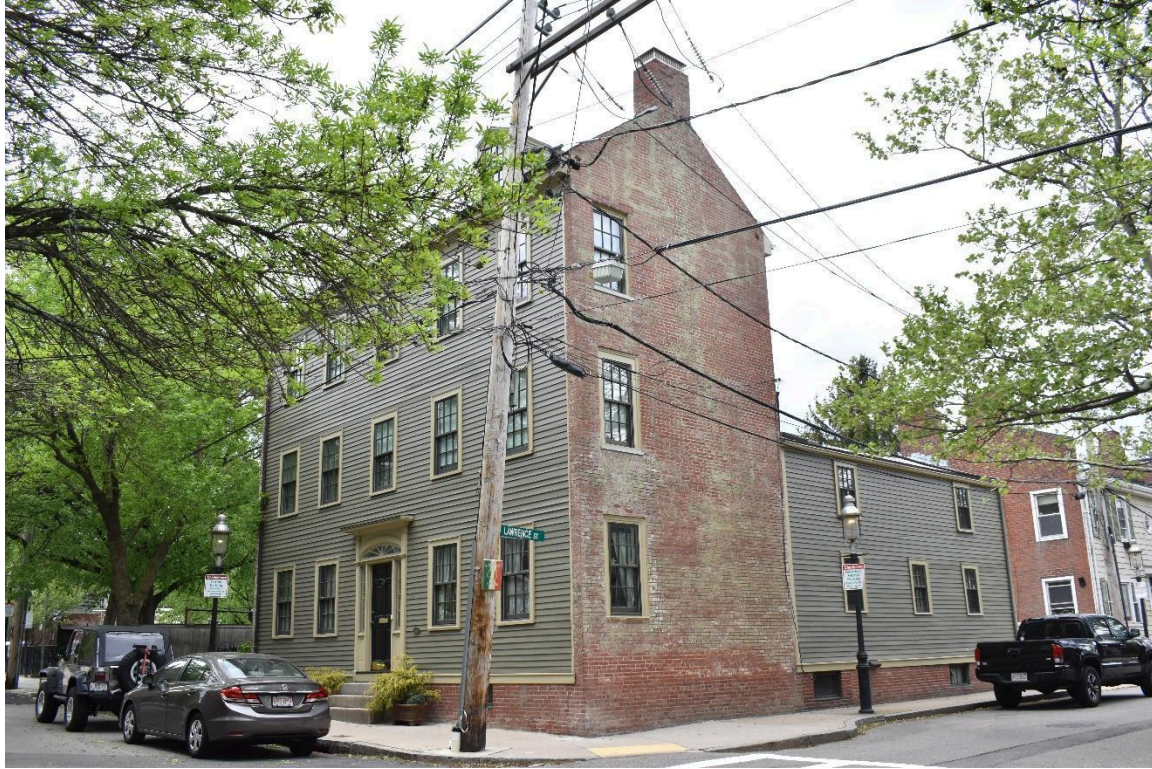
Figure 5. South and east elevations, looking northwest, 8 Lawrence St. at right. Photo by The Public Archaeology Laboratory, Inc.
