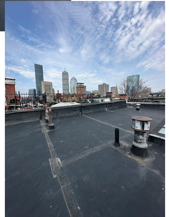
Existing parapet on North side party wall. (2-3' above roof)
