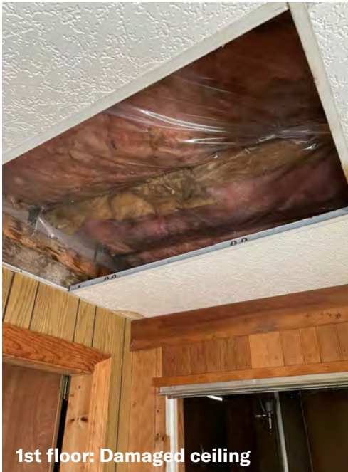
1st floor: damaged ceiling, water leakage
