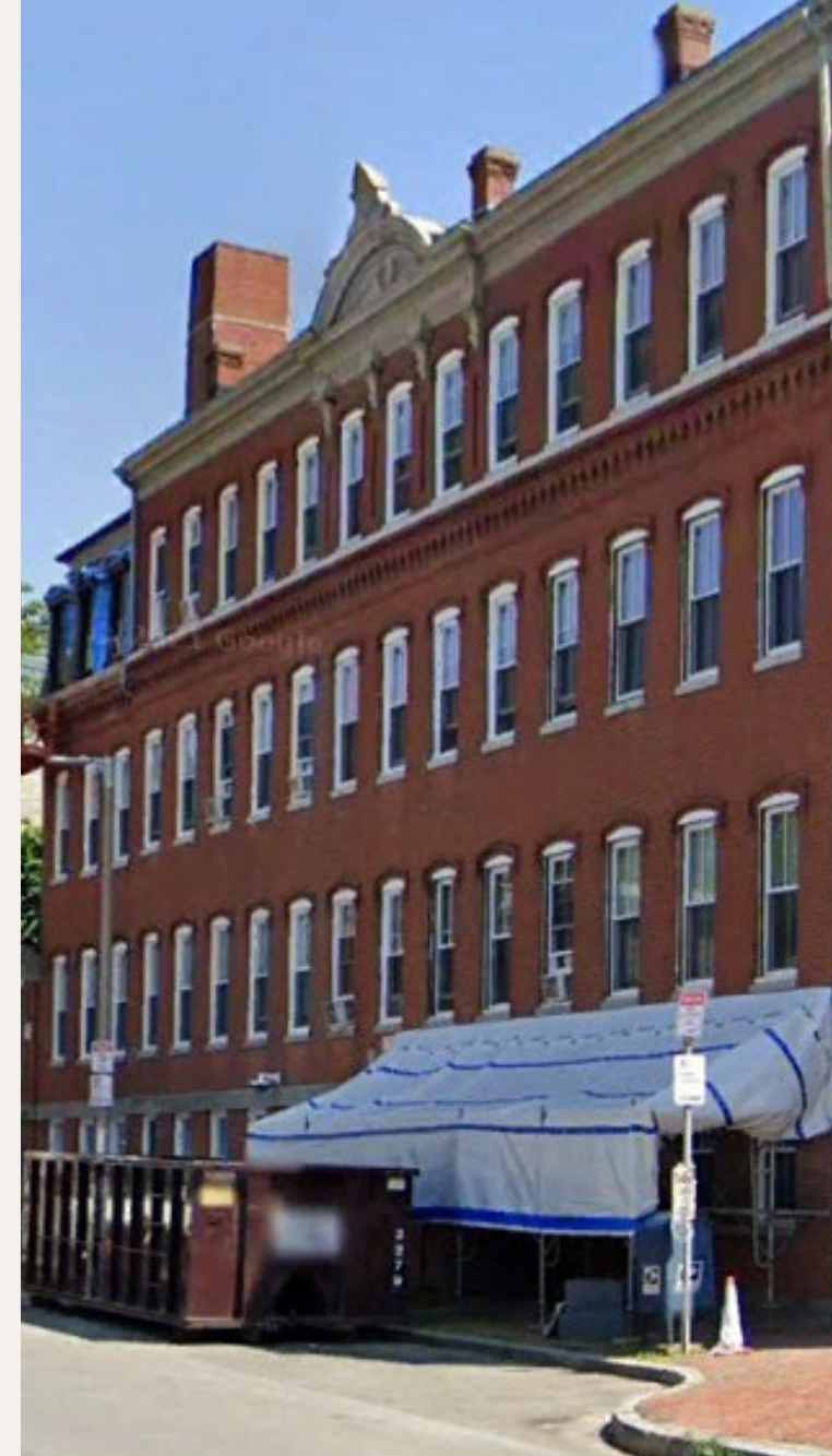
3. 286 Roxbury Street (Adjacent Building)
