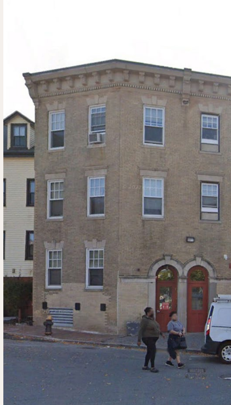
2. 288-300 Roxbury Street (ACD Historically Significant)
