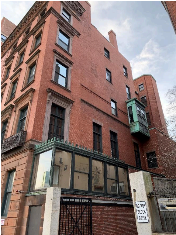
Figure 3. East elevation. Photo by Martha Brest (March 25, 2024).
