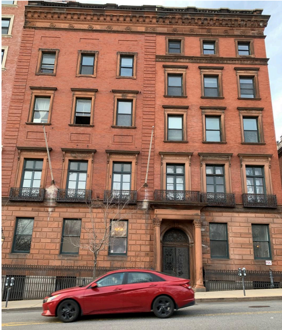
Figure 2. South façade. Photo by Martha Brest (March 25, 2024).
