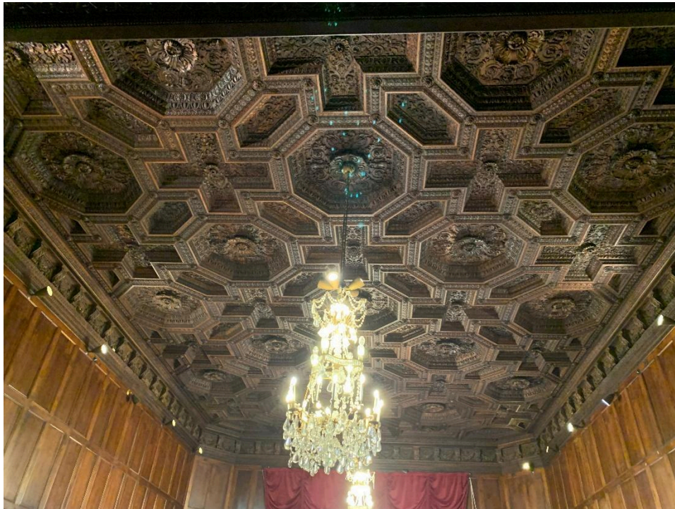
Figure 14. Second floor, Music Room ceiling. Photo by Martha Brest (August 21, 2023).
