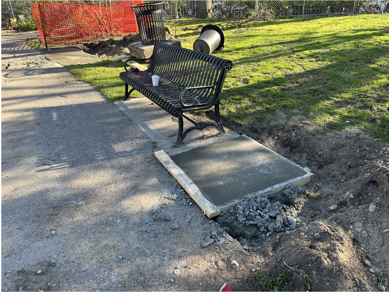
ADA Companion seating along the central walkway has been installed. SITE PHOTO 4/16/24
