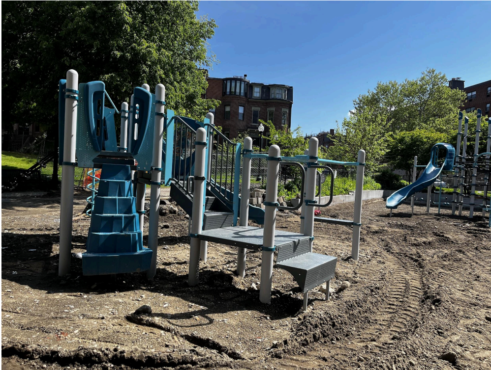
The 2-5 play equipment has been installed! SITE PHOTO 5/17/24
