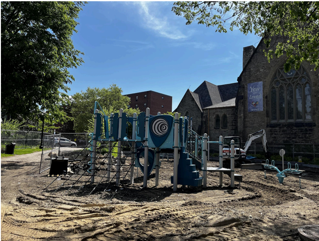
The 5-12 play equipment has been installed! SITE PHOTO 5/17/24
