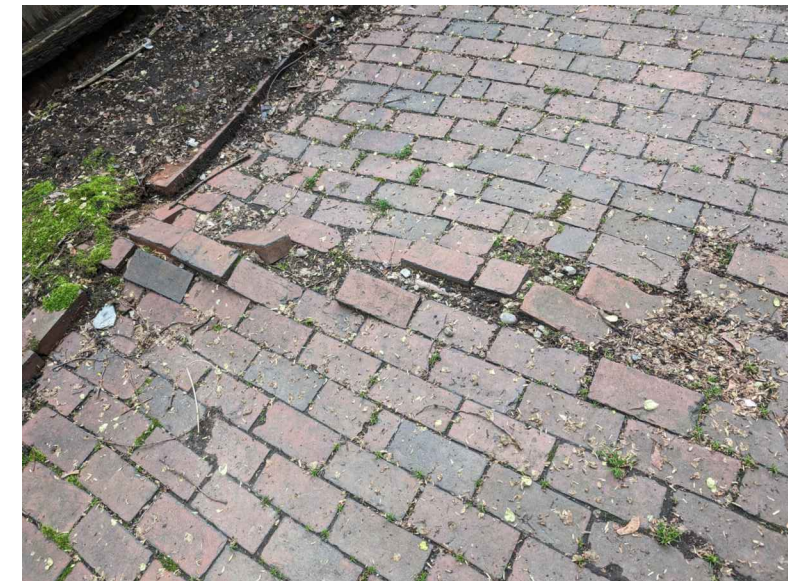
VIEW OF REAR YARD SHOWING TREE ROOTS DISPLACING PAVERS
