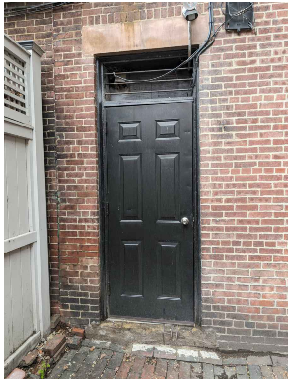
VIEW OF EXISTING COMMON EGRESS DOOR
