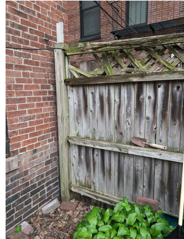
VIEW OF EXISTING PERIMETER FENCE
