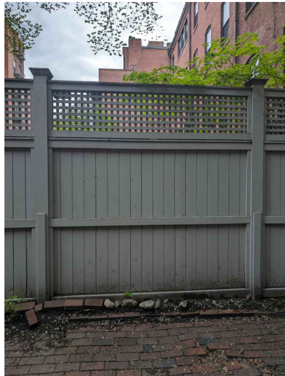
VIEW OF EXISTING FENCE AT 338 MARLBORO ST.
