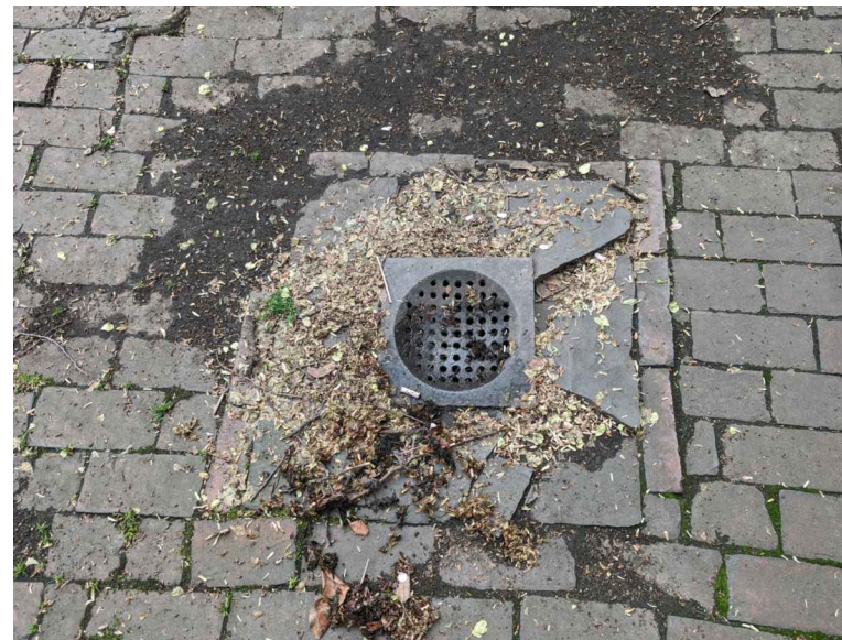
VIEW OF REAR YARD SHOWING EXISTING SITE DRAIN
