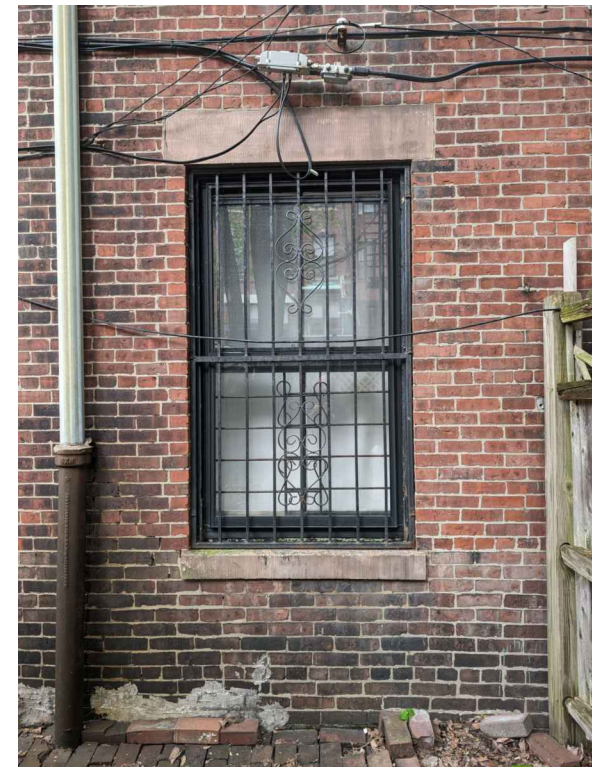
VIEW OF EXISTING WINDOW TO REMAIN
