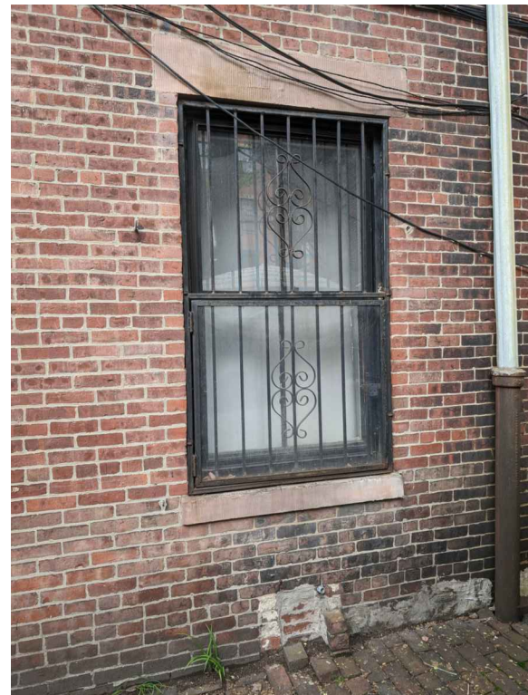
VIEW OF EXISTING WINDOW PROPOSED TO BE REMOVED
