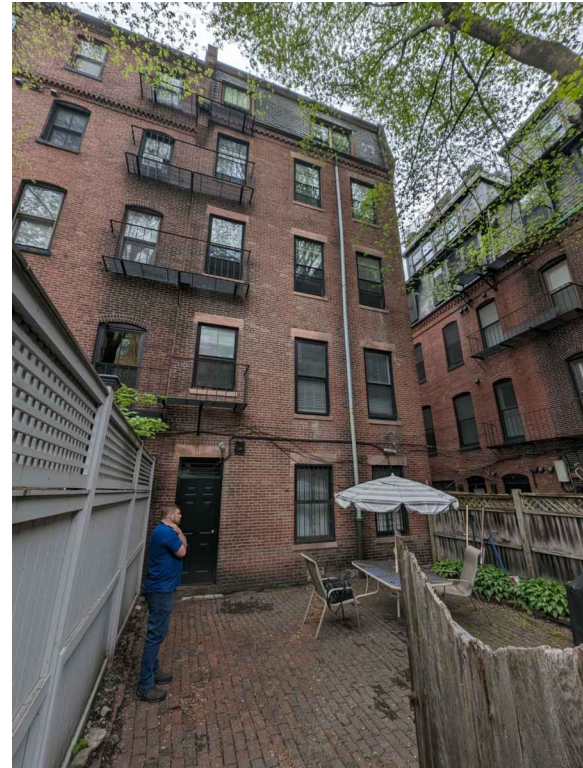
VIEW OF REAR YARD FROM GATE
