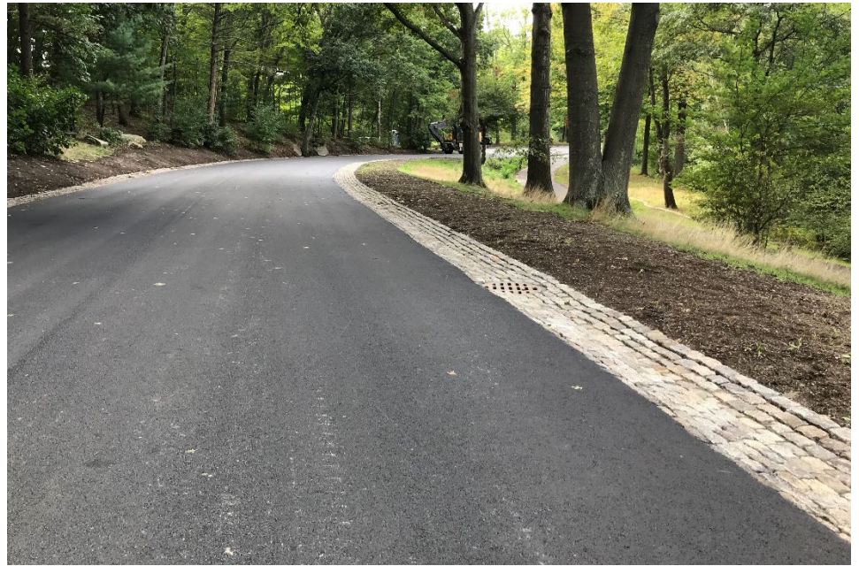
COBBLE SWALE / SLOPE TO PREVENT EROSION
