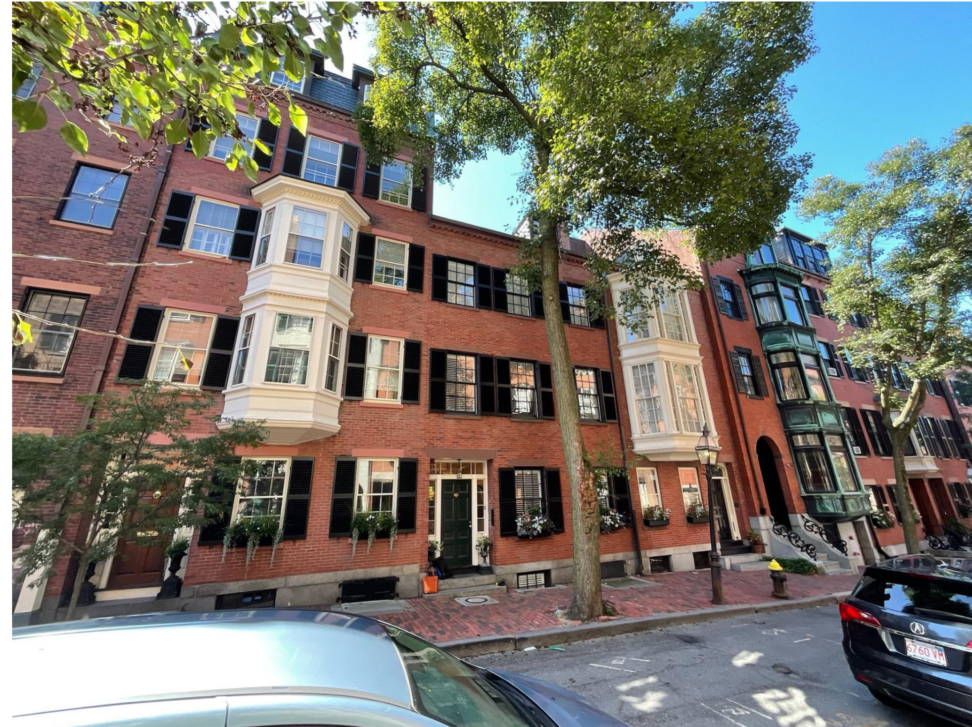
EXISTING PUBLIC STREET VIEW
