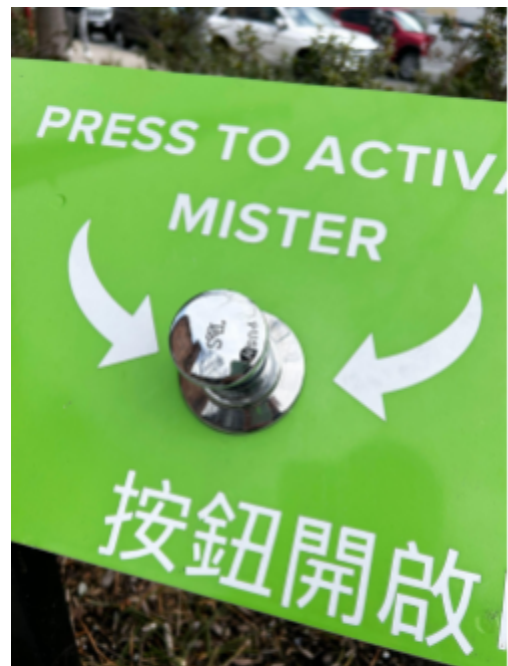
Example of a metered water valve. This type of valve is set to dispense water for a defined amount of time, meaning there is no risk of water being left on.
