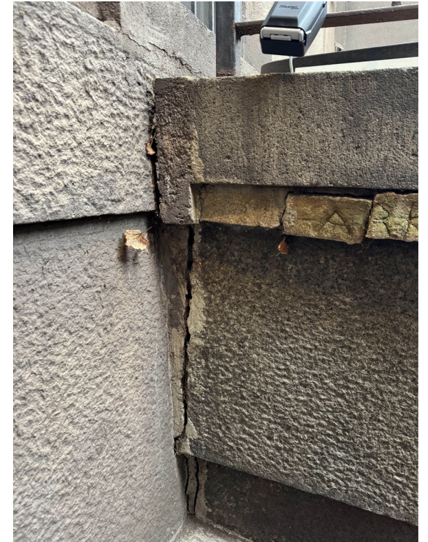
VIEW FROM BELOW (GARDEN LEVEL ENTRY) RETAINING WALL COLLAPSE / BUILDING FOUNDATION DAMAGE CAUSED BY OVERGROWN TREE ROOT SYSTEM
