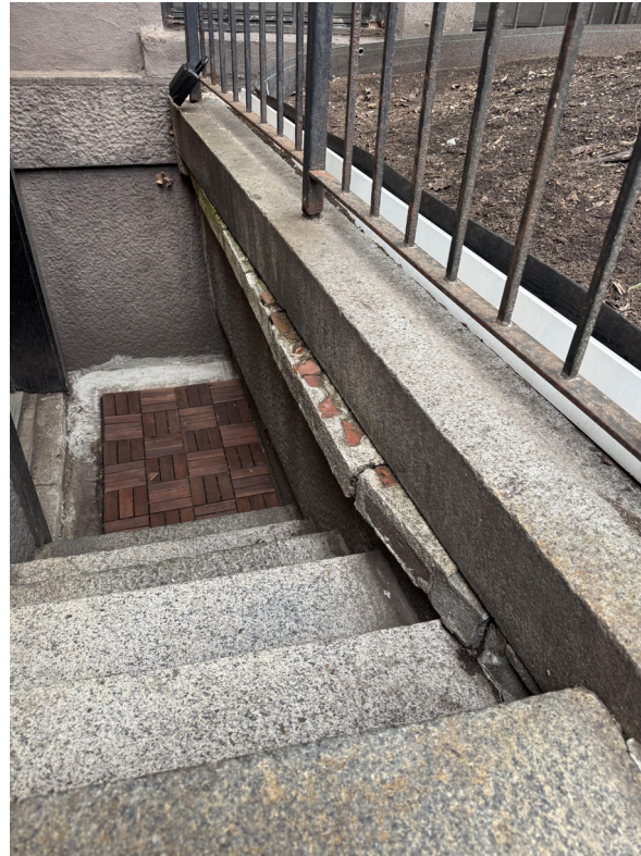
VIEW FROM SIDEWALK RETAINING WALL COLLAPSE CAUSED BY OVERGROWN TREE ROOT SYSTEM
