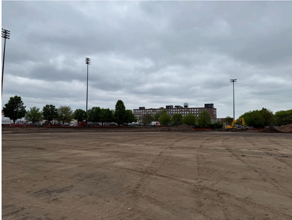
Topsoil stripping
