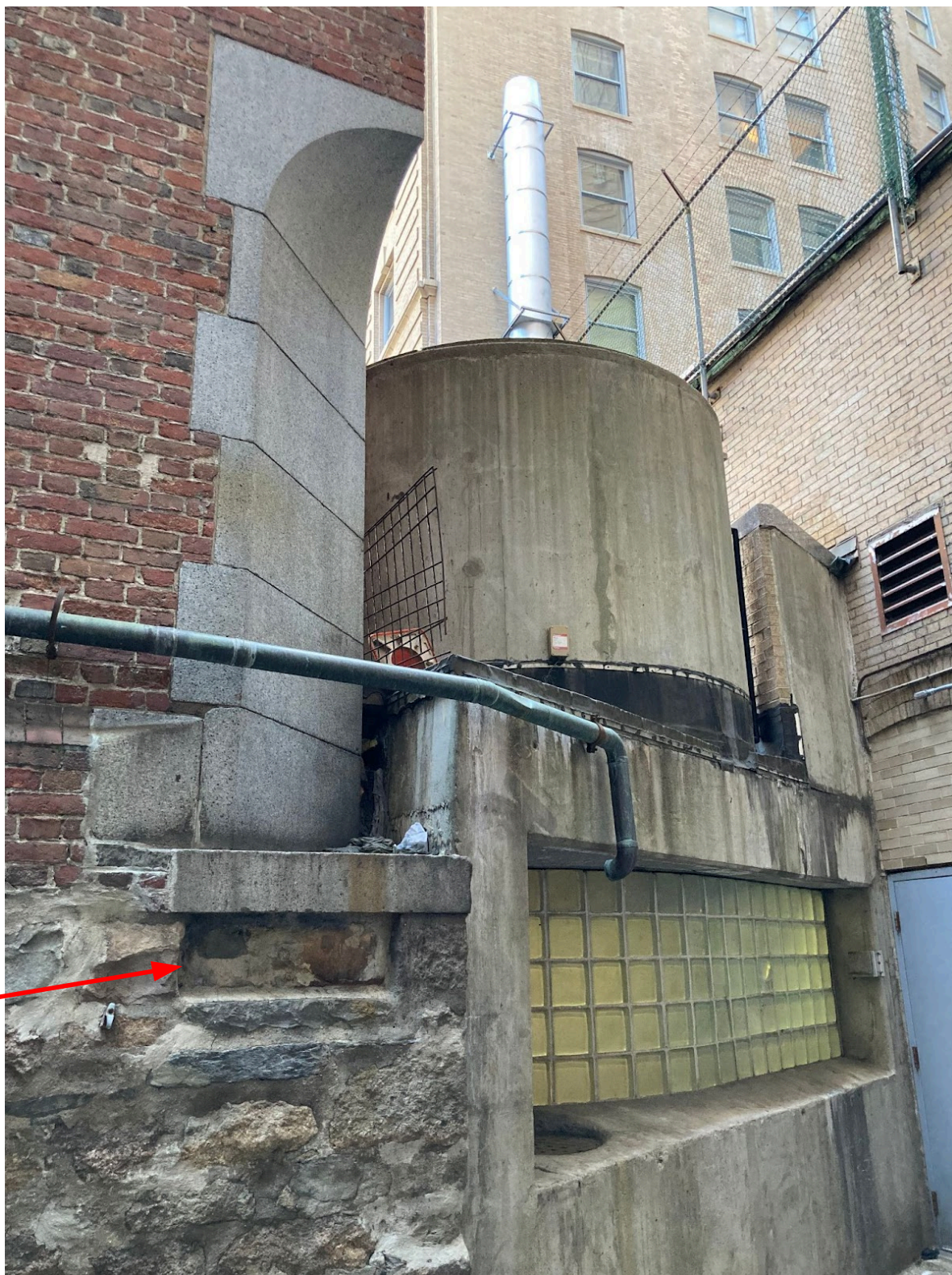
Photo 4. The northeast corner of the Old South Meeting House, where part of the brick facade was removed and capped with granite to make room for alterations at the adjacent MBTA State Street T station in the 1980s. The cornerstone carved with “JB 1729” is indicated by the red arrow (J. Gaugler, photographer, April 2025).
