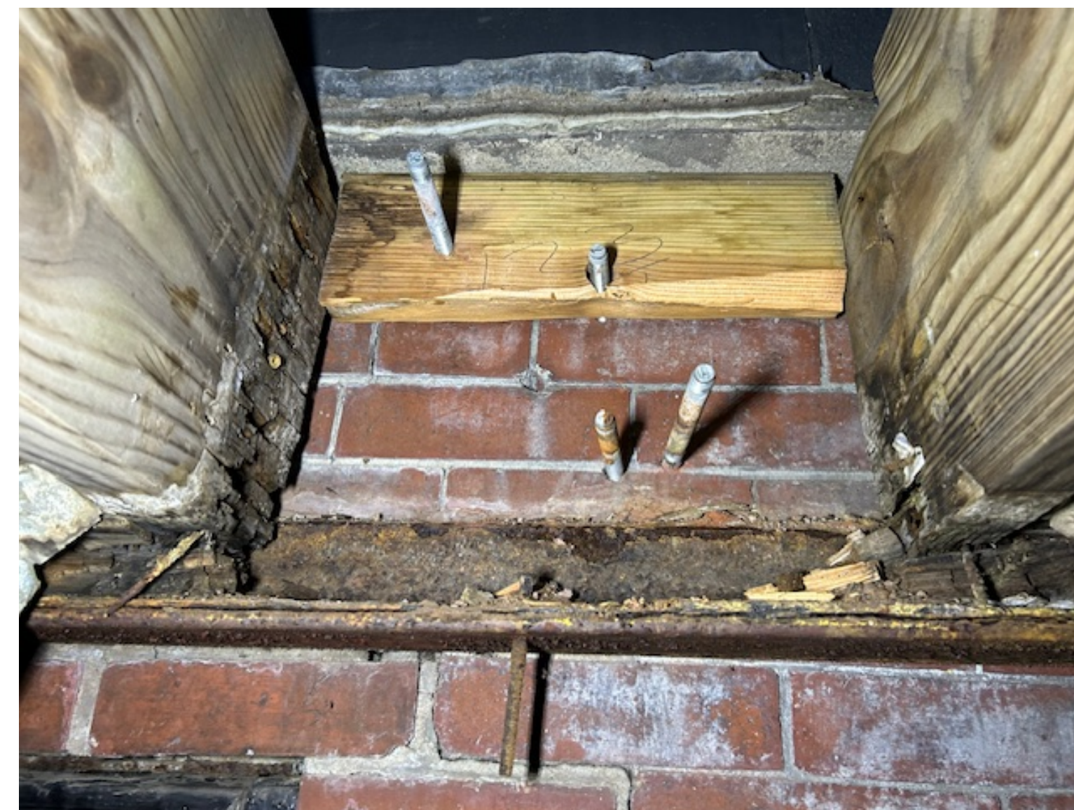
Underside of joists, showing rot
