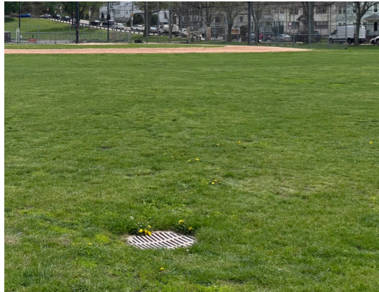
1 Grades pitch toward center of field, causes ponding
