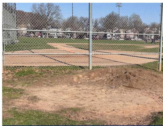
3 Infield sand washing out over worn down edges
