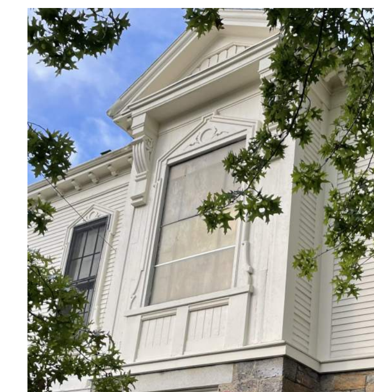
Window Trim Detail
