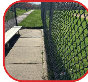
WARPED FENCE
