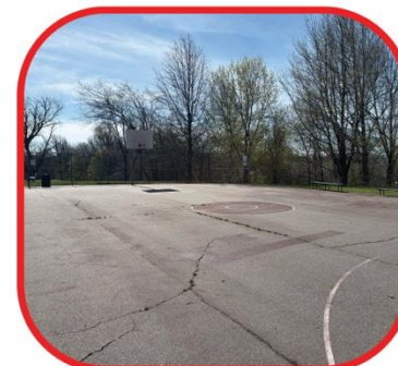
CRACKED ASPHALT
