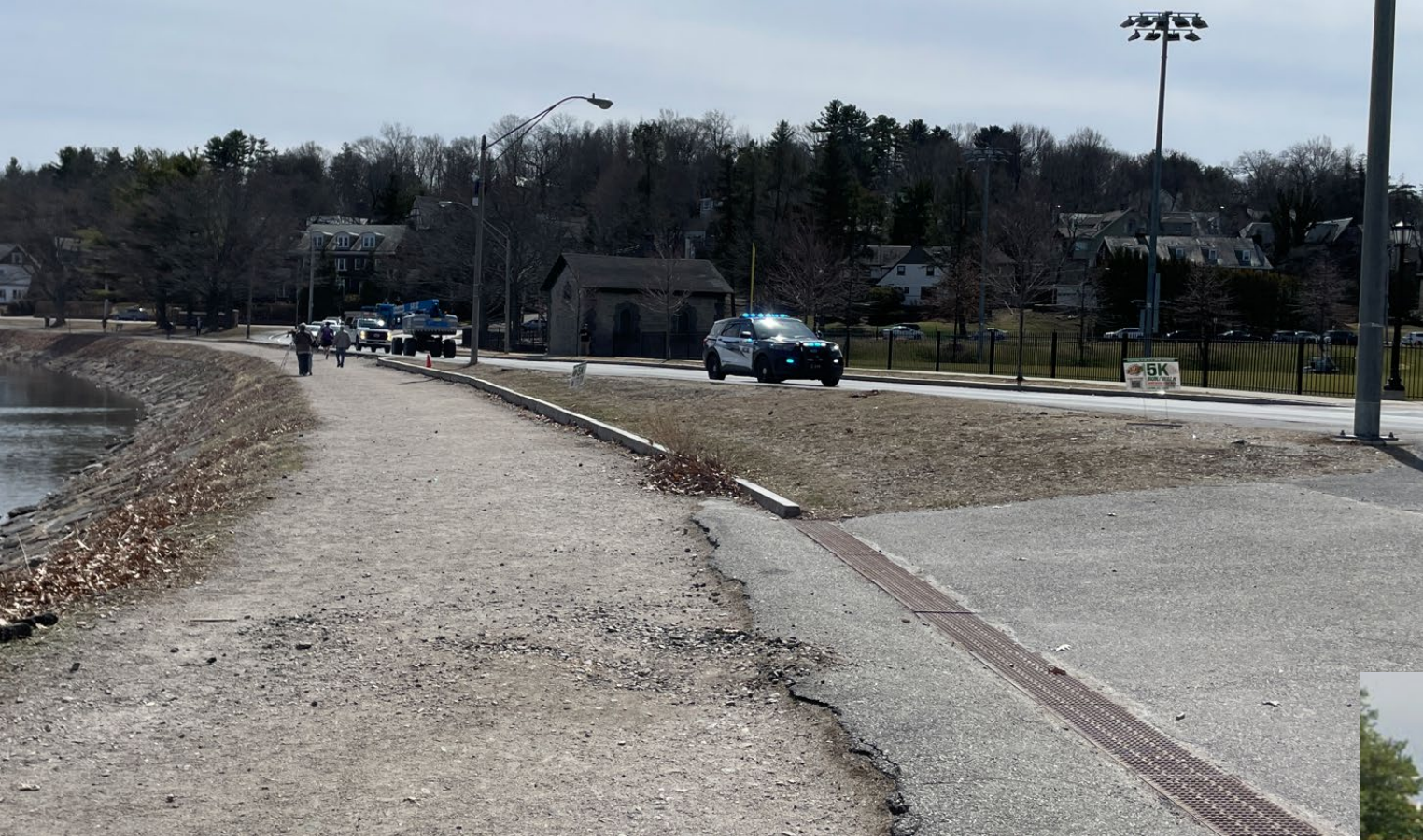
Views of existing granite curbing and narrow grated slot drain just north of project area along Chestnut Hill Driveway
