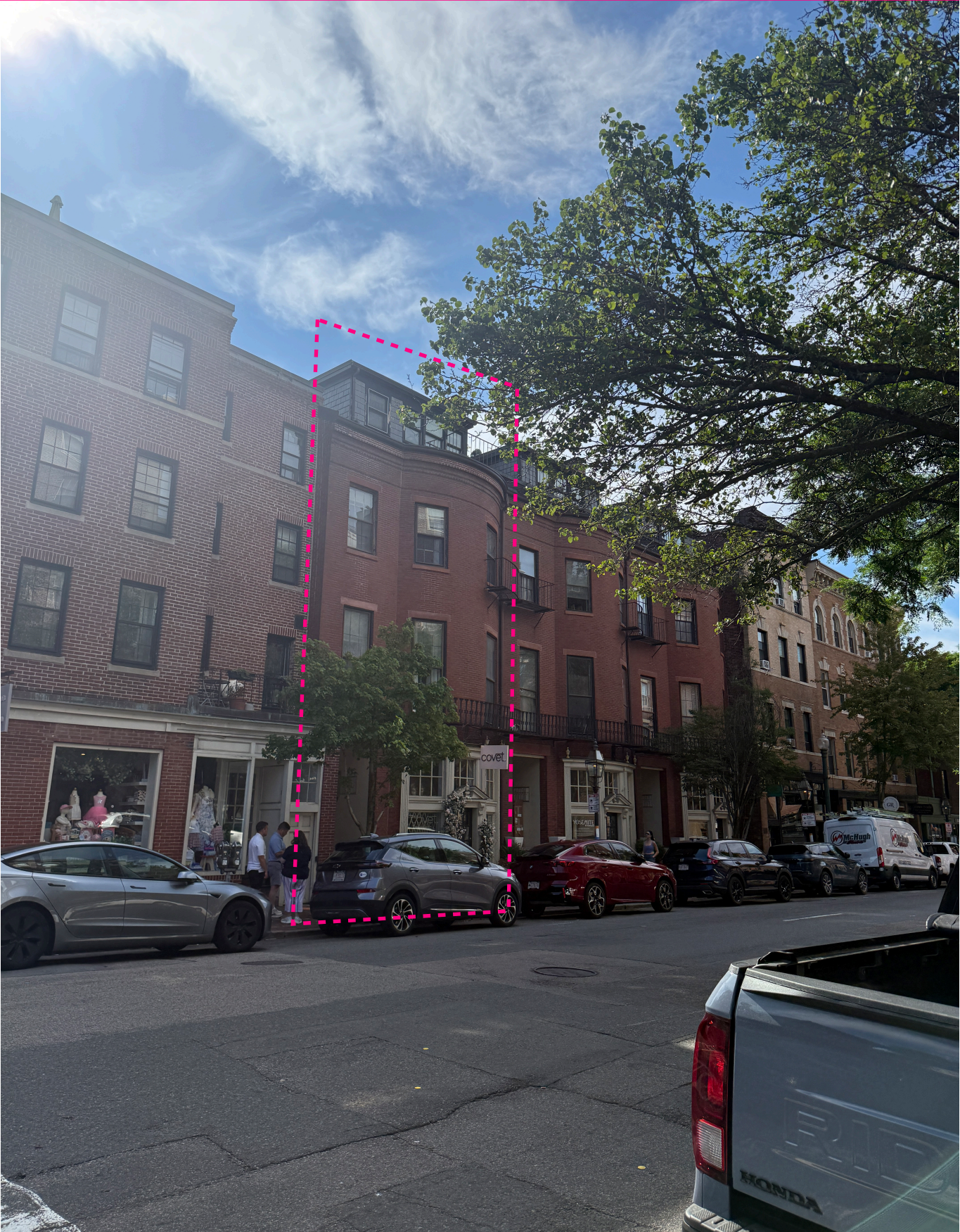
SOUTH EAST VIEW AT CHARLES ST & REVERE ST
