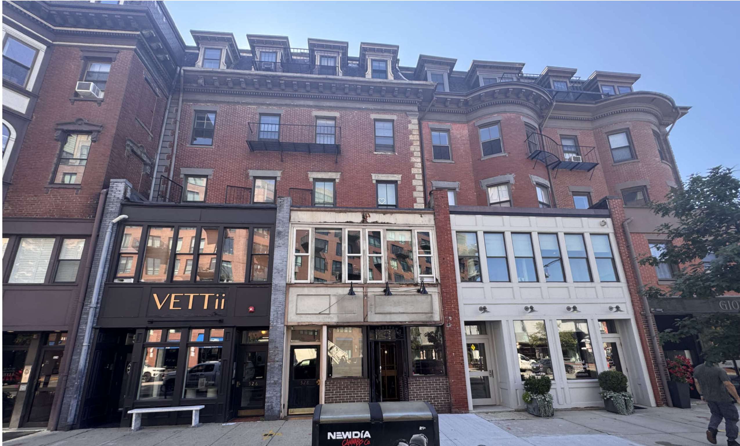
FRONT ELEVATION PHOTO – EXISTING
