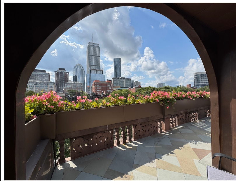
EXISTING CONDITIONS PHOTO 2
