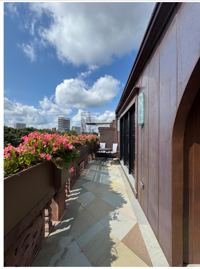
EXISTING CONDITIONS PHOTO 1
