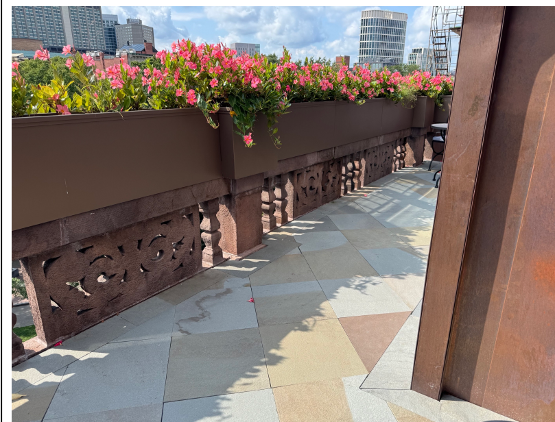
EXISTING CONDITIONS PHOTO 3
