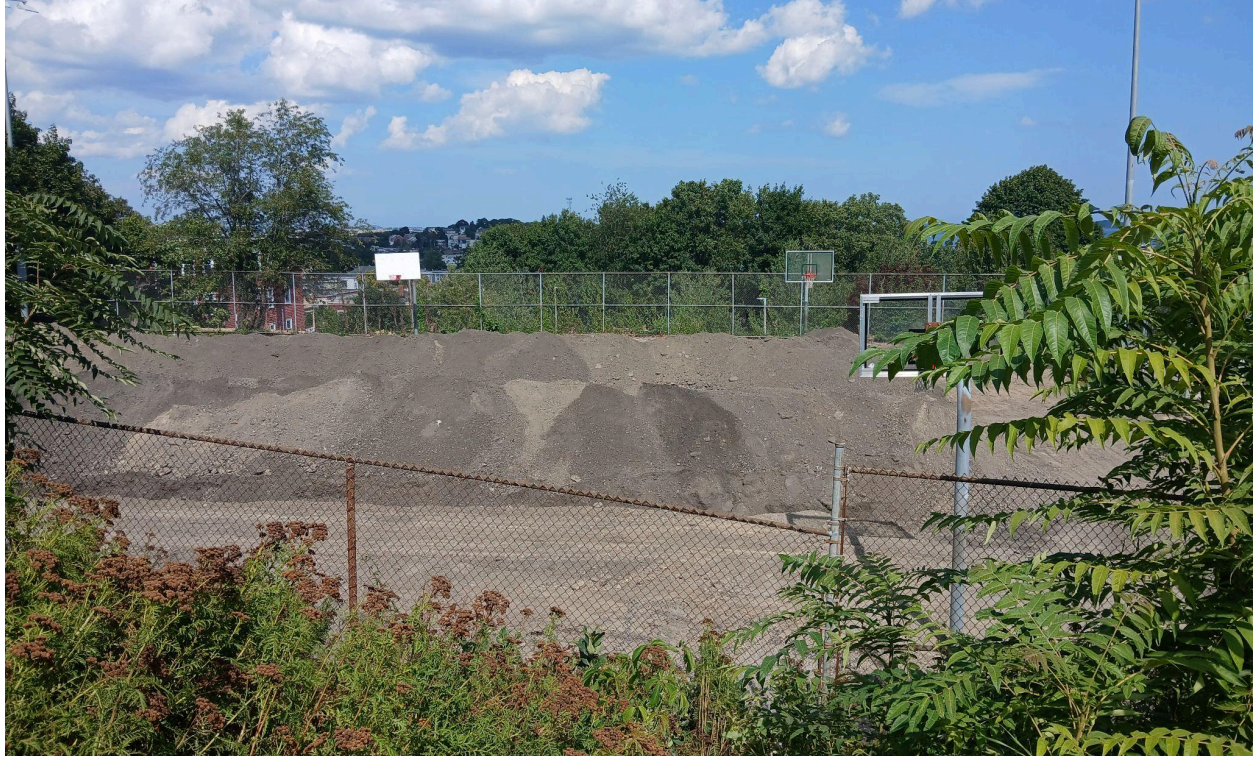
Basketball court pavement demolition as seen from the former stair.
