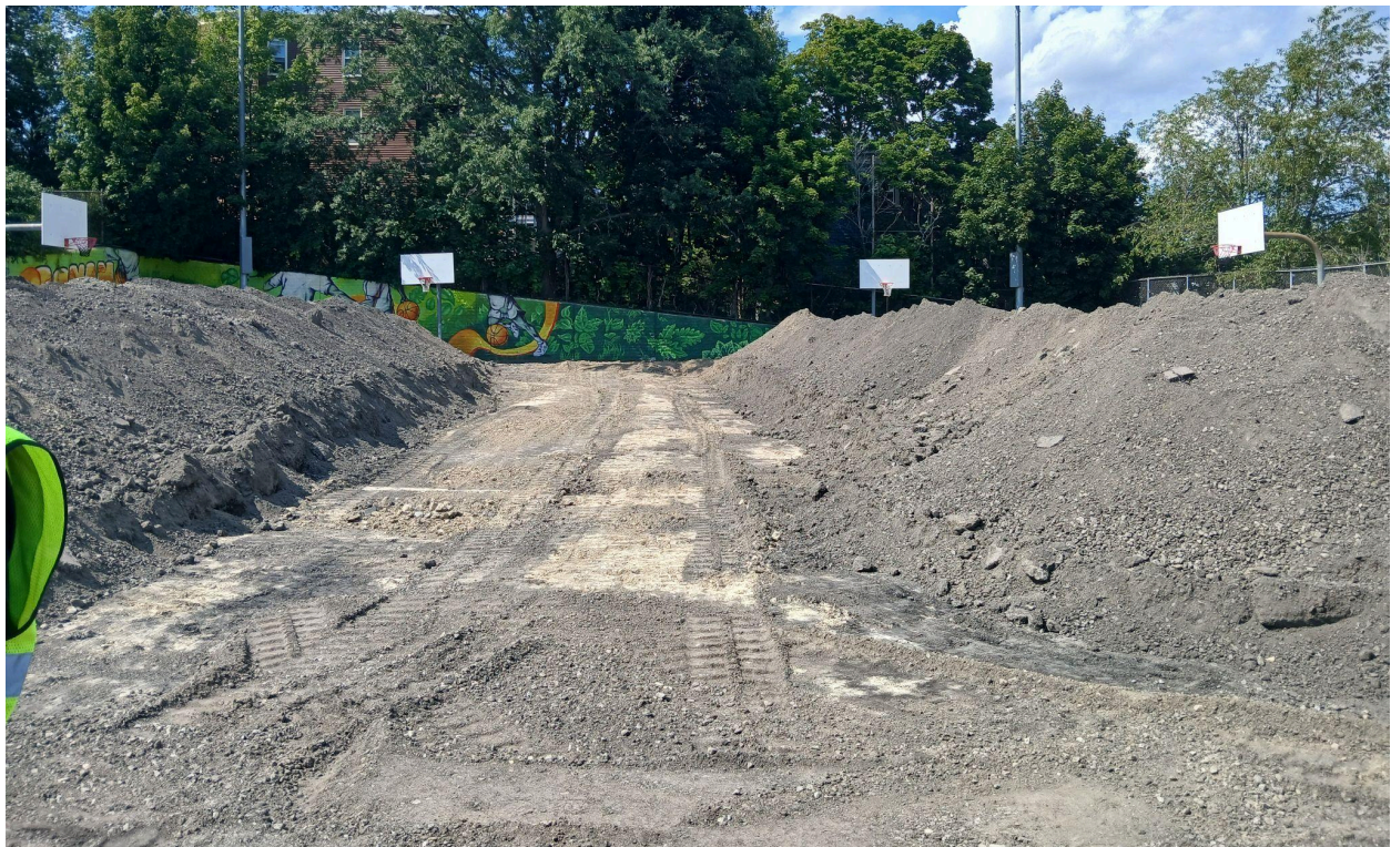
Basketball court pavement demolition with view of protected mural beyond.
