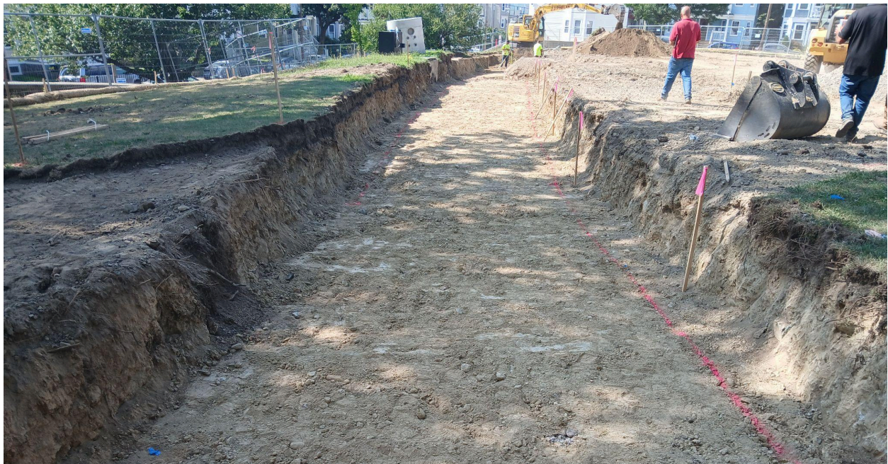
Excavation for new porous asphalt pathway loop.
