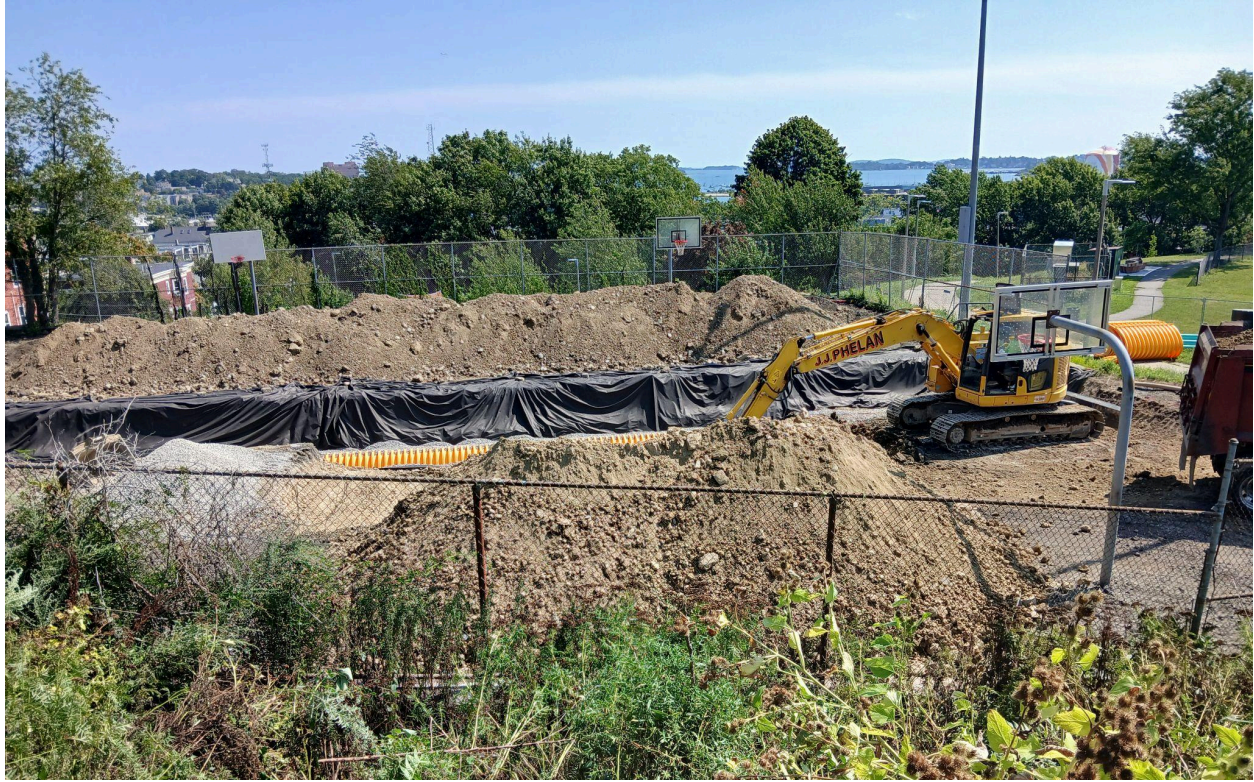
Basketball court drainage infrastructure being installed.
