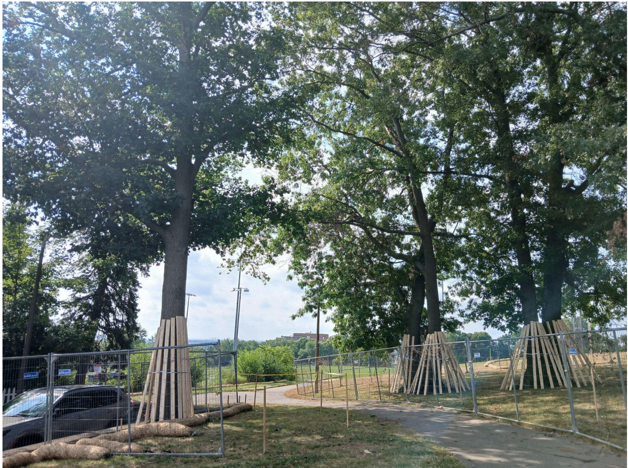
Tree protection measures.
