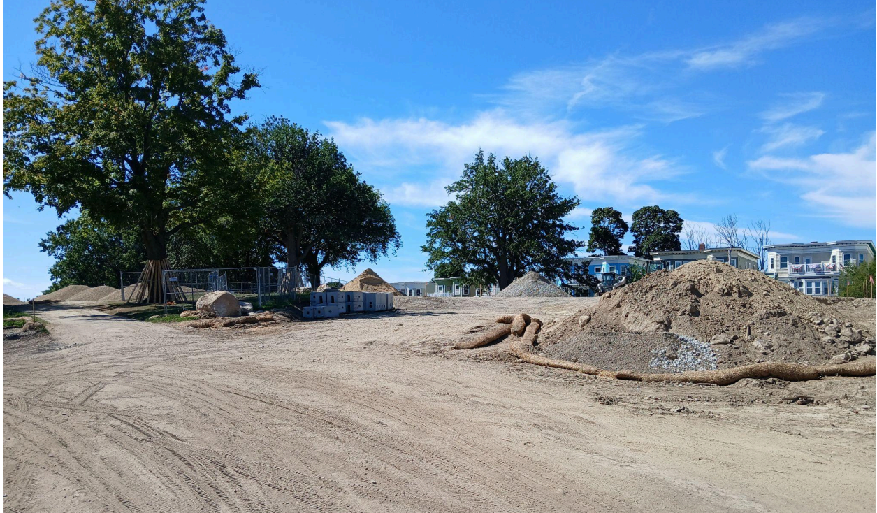
A view into the site from the vehicular entrance at Marie Street. The contractor uses a watering truck to spray down the ground and piles each day to prevent dust in the air.
