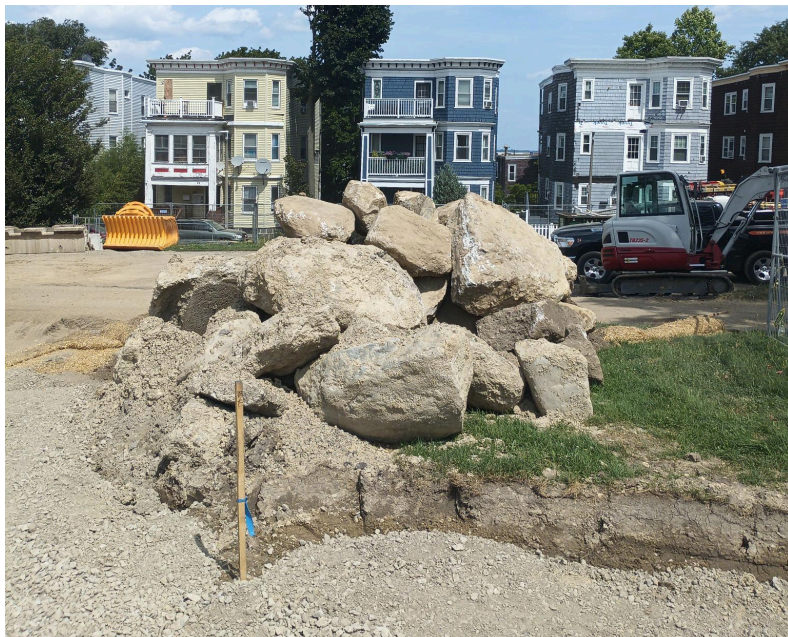
Some of the boulders that have been uncovered and collected during excavation, which will be incorporated into the renovation in various ways.
