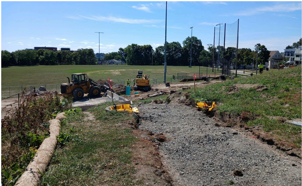
View down from the top of the former staircase to where more drainage infrastructure is being installed.
