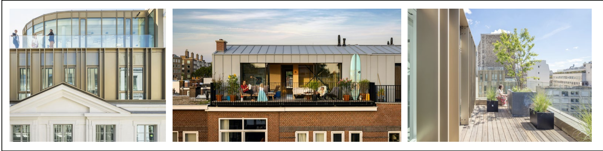
Light toned rooftop cladding
