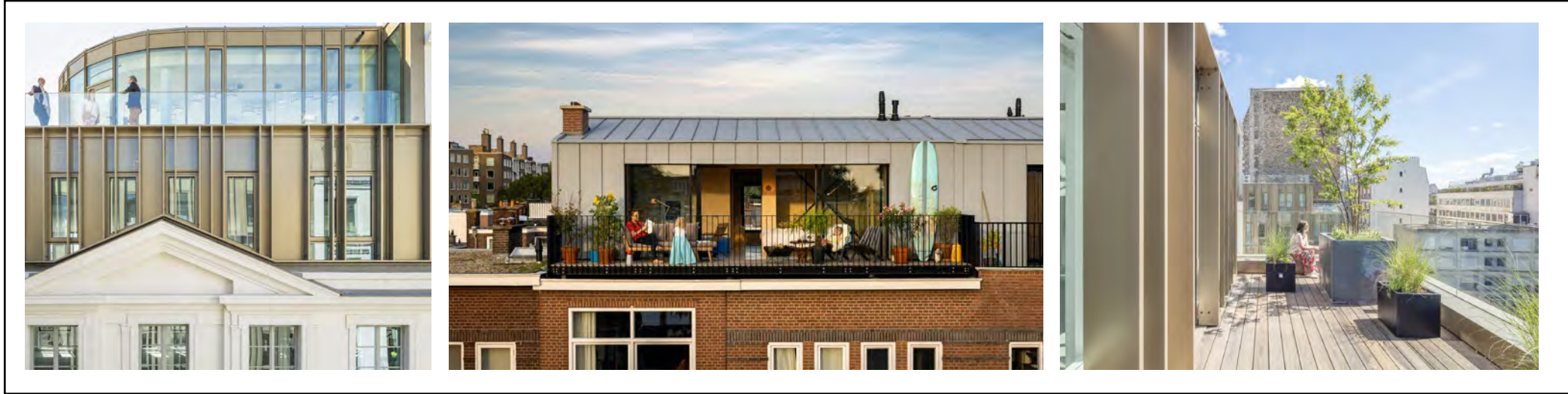
Light toned rooftop cladding
