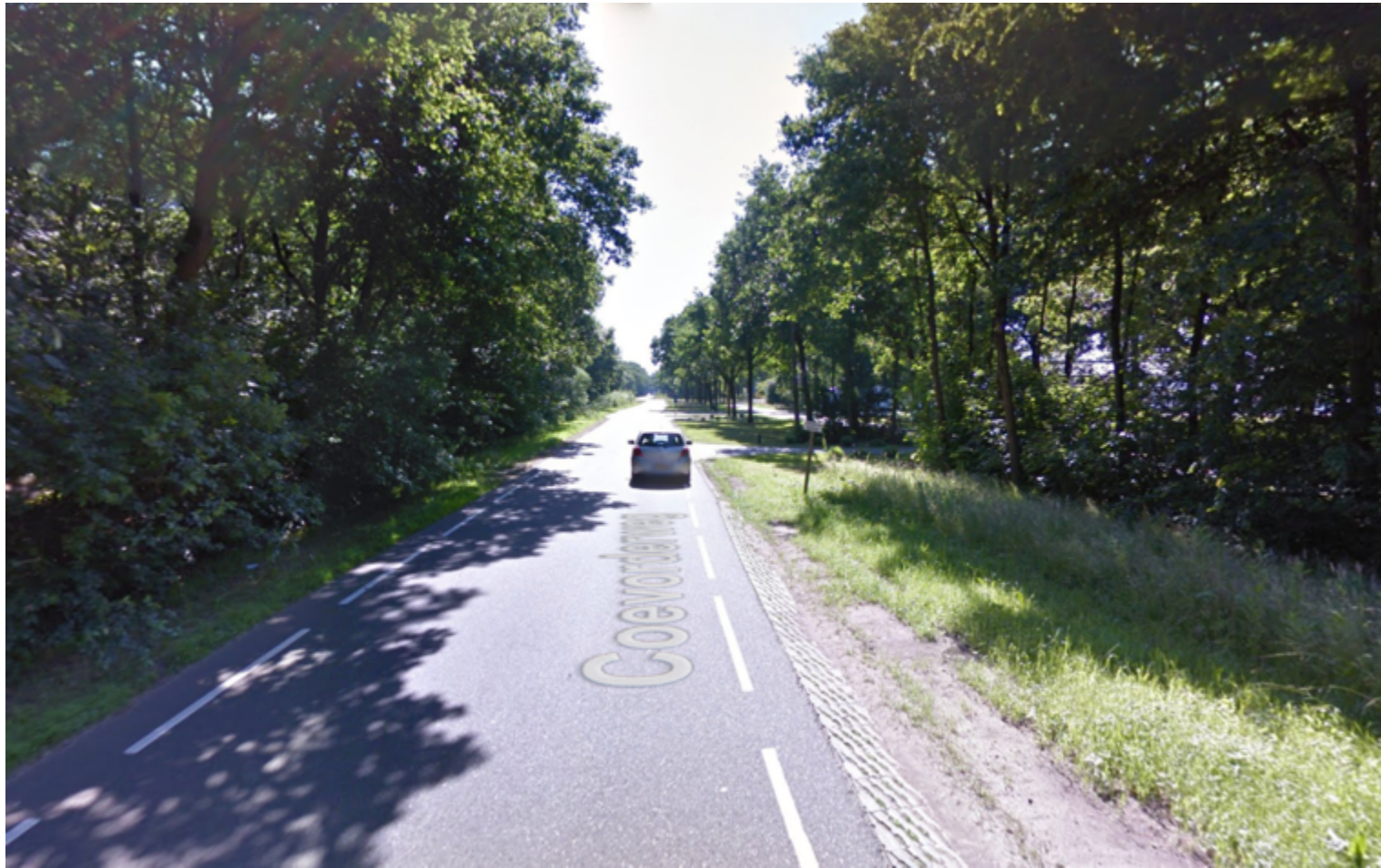
Rural Road after implementation 60 km/h zone (2016)
