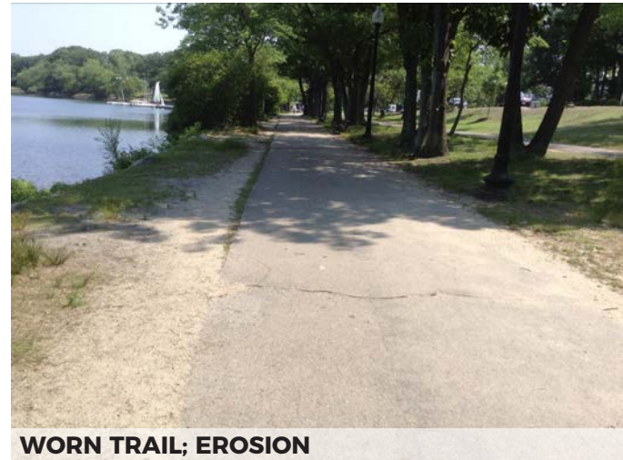
WORN TRAIL; EROSION
