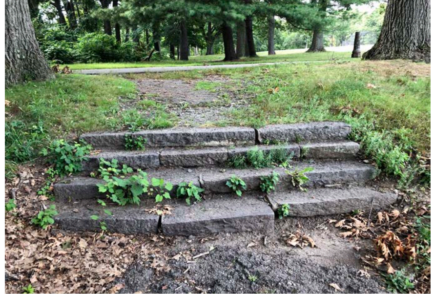
EXISTING STAIR TREADS
