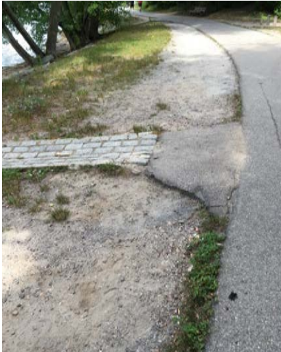
WORN TRAIL; EROSION
