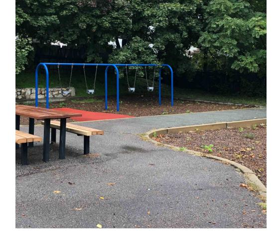
Concrete curbs are located between paths, lawn, and existing play areas with +/- 6 inch difference in elevation. All walkways and picnic area are asphalt.
